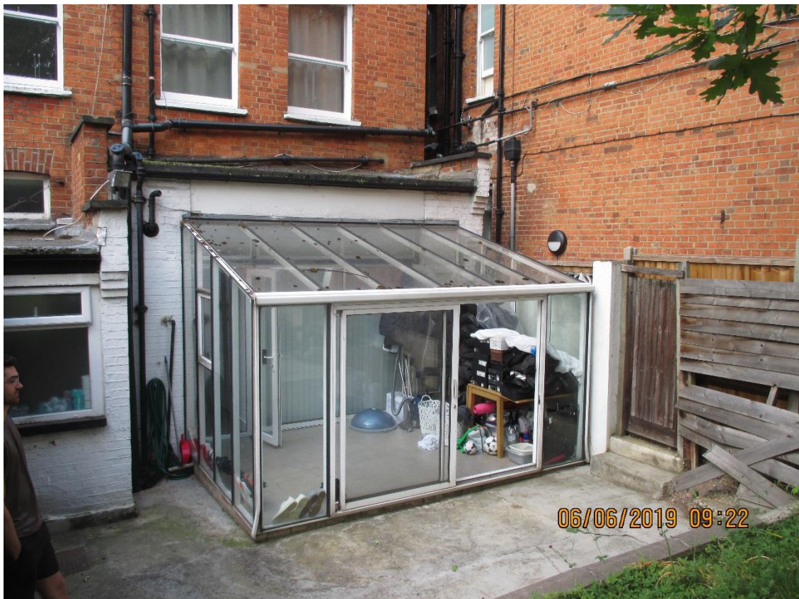
Existing conservatory to be demolished
