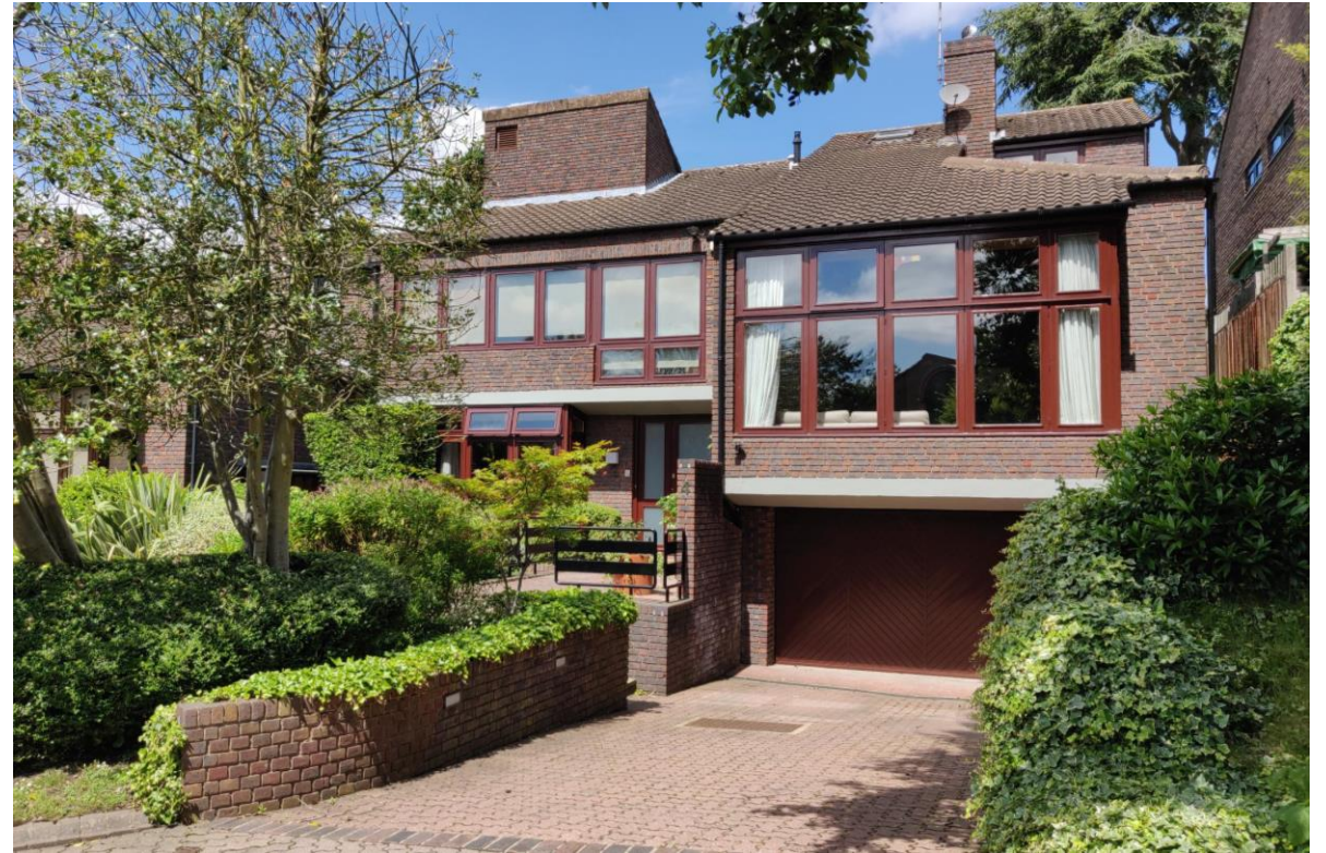
PHOTOGRAPH OF EXISTING FRONT ELEVATION
