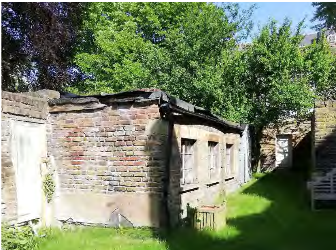
Photo 7, Outbuilding on 20 Perrins Cottage Side
