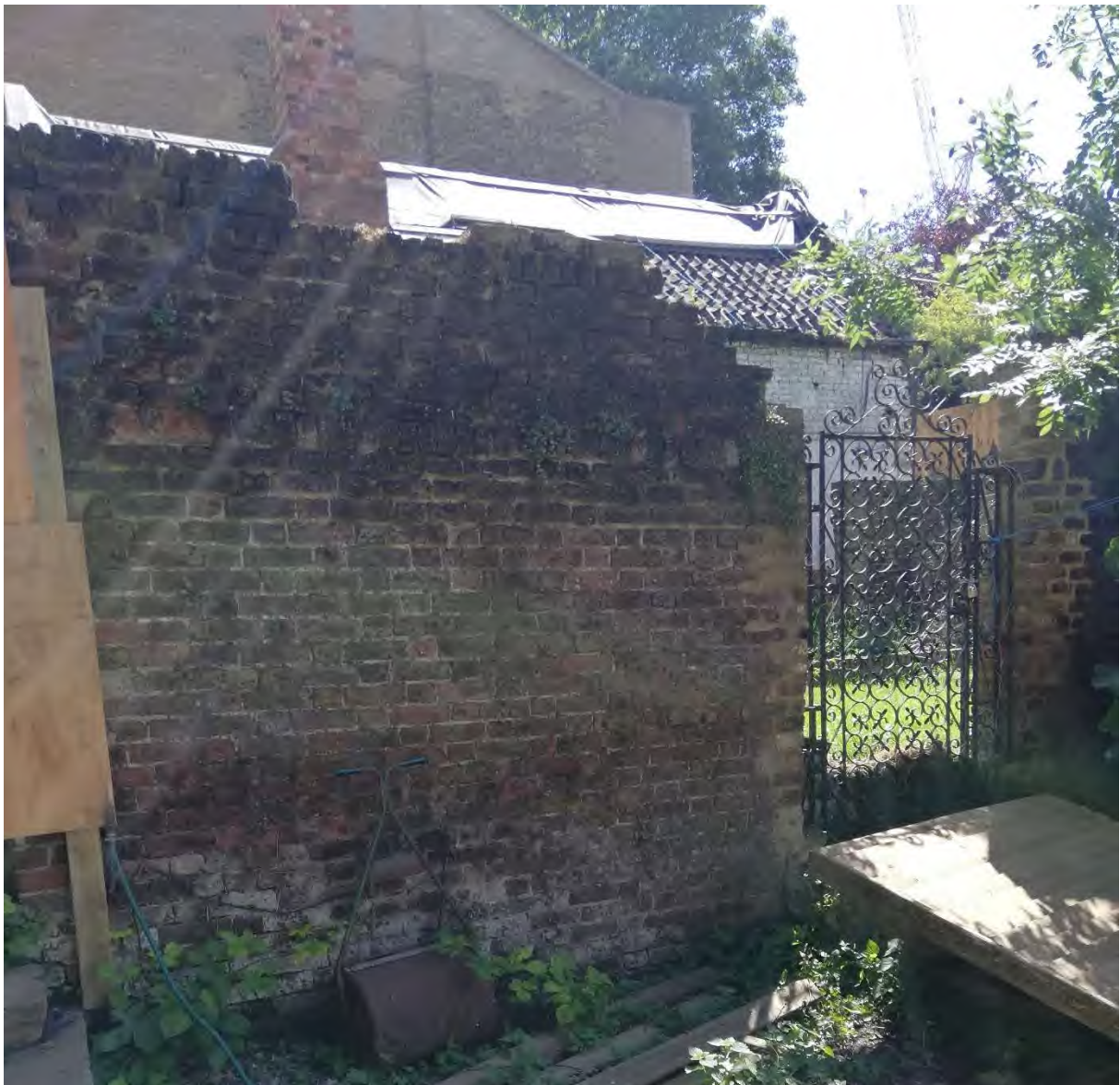
Photo 12, Elevation 4, LHS of opening 1 on 22 Frognal Way side
