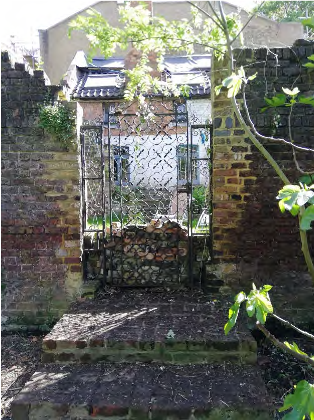
Photo 15, Opening 1 with new brickwork evident
