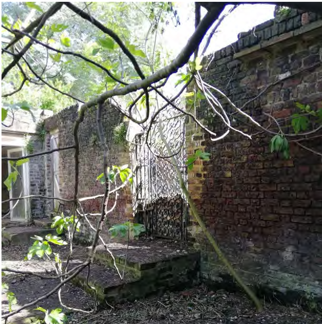
Photo 14, Opening 1 in foreground with Opening 2 & Outbuilding in background
