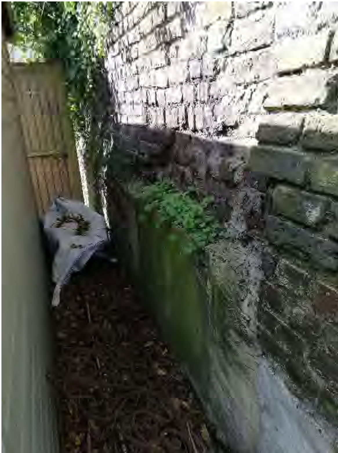
Photo 2, Southern section of wall behind existing shed
