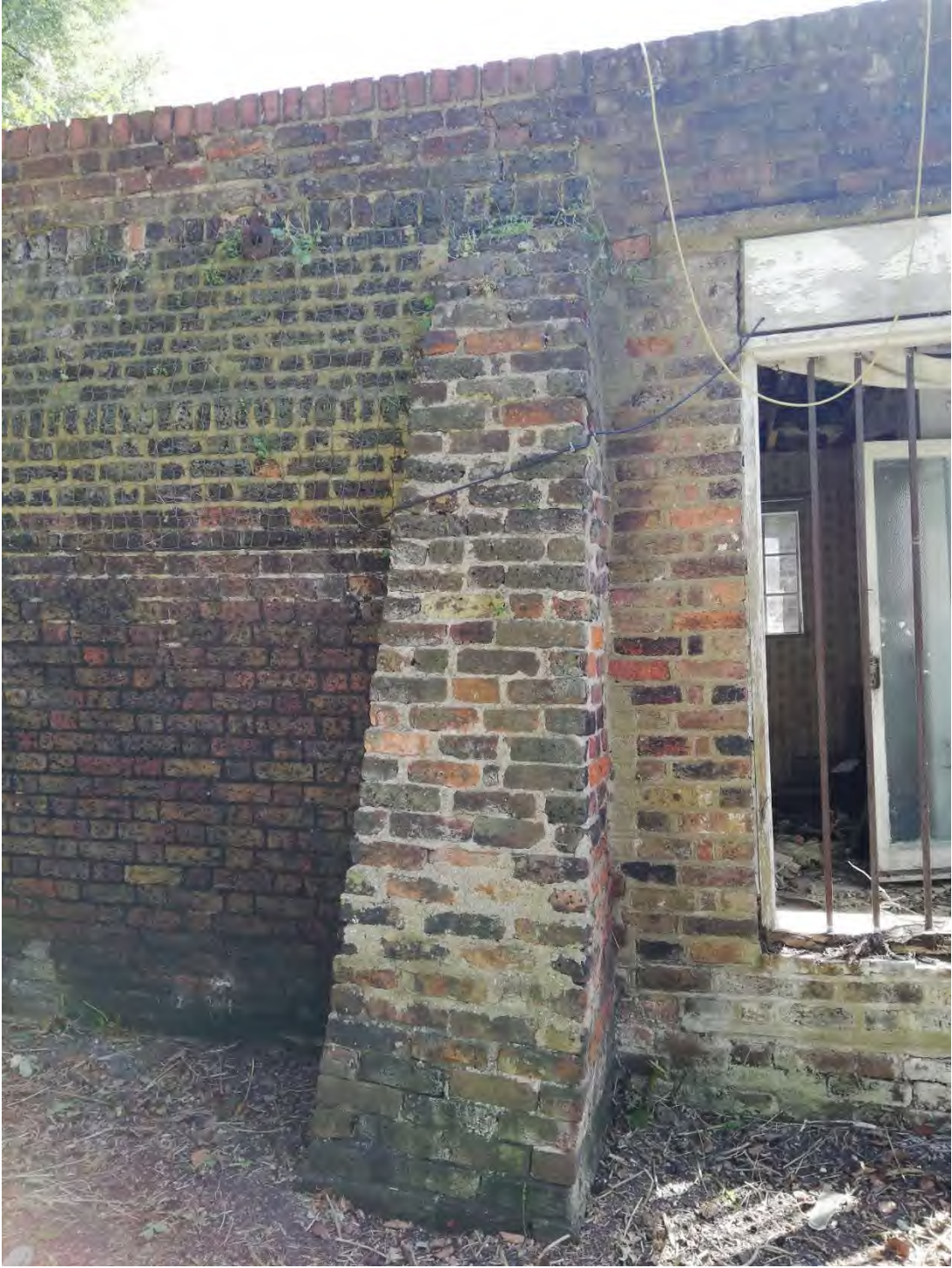
Photo 10, Right-hand side masonry pier to Outbuilding
