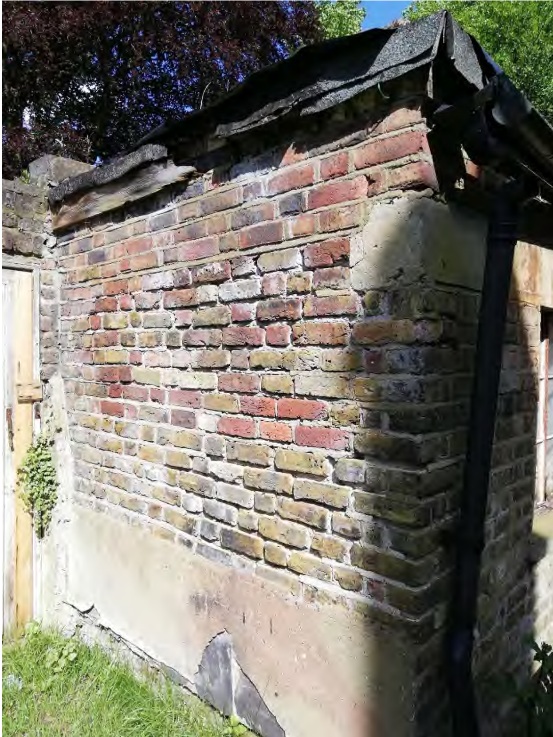
Photo 8, View of Outbuilding Masonry
