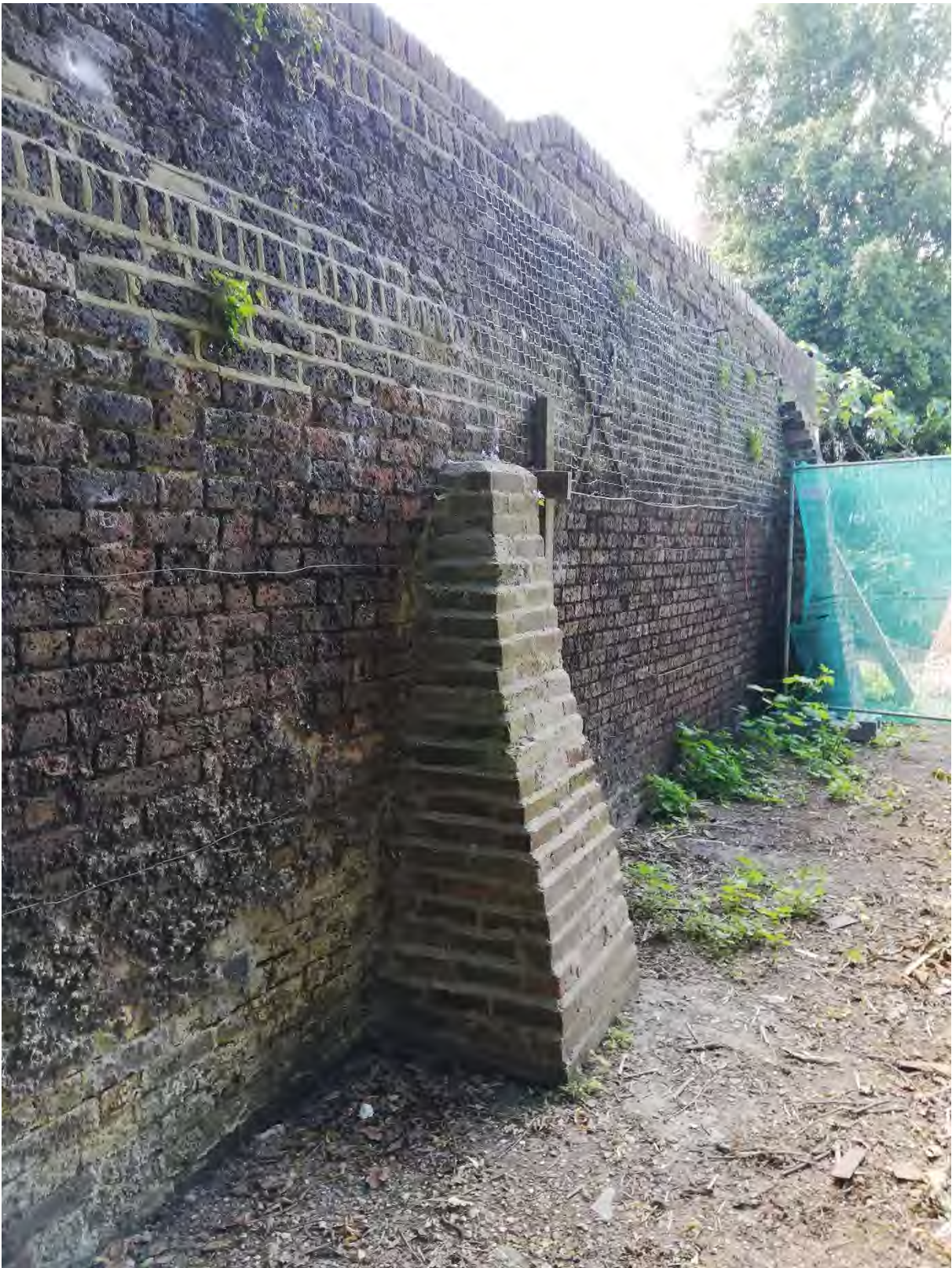
Photo 9, North section of wall and viewing toward the into Outbuilding entrance
