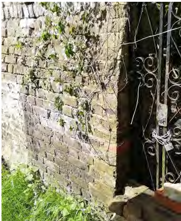
Photo 5, new/old brickwork at opening reveal
