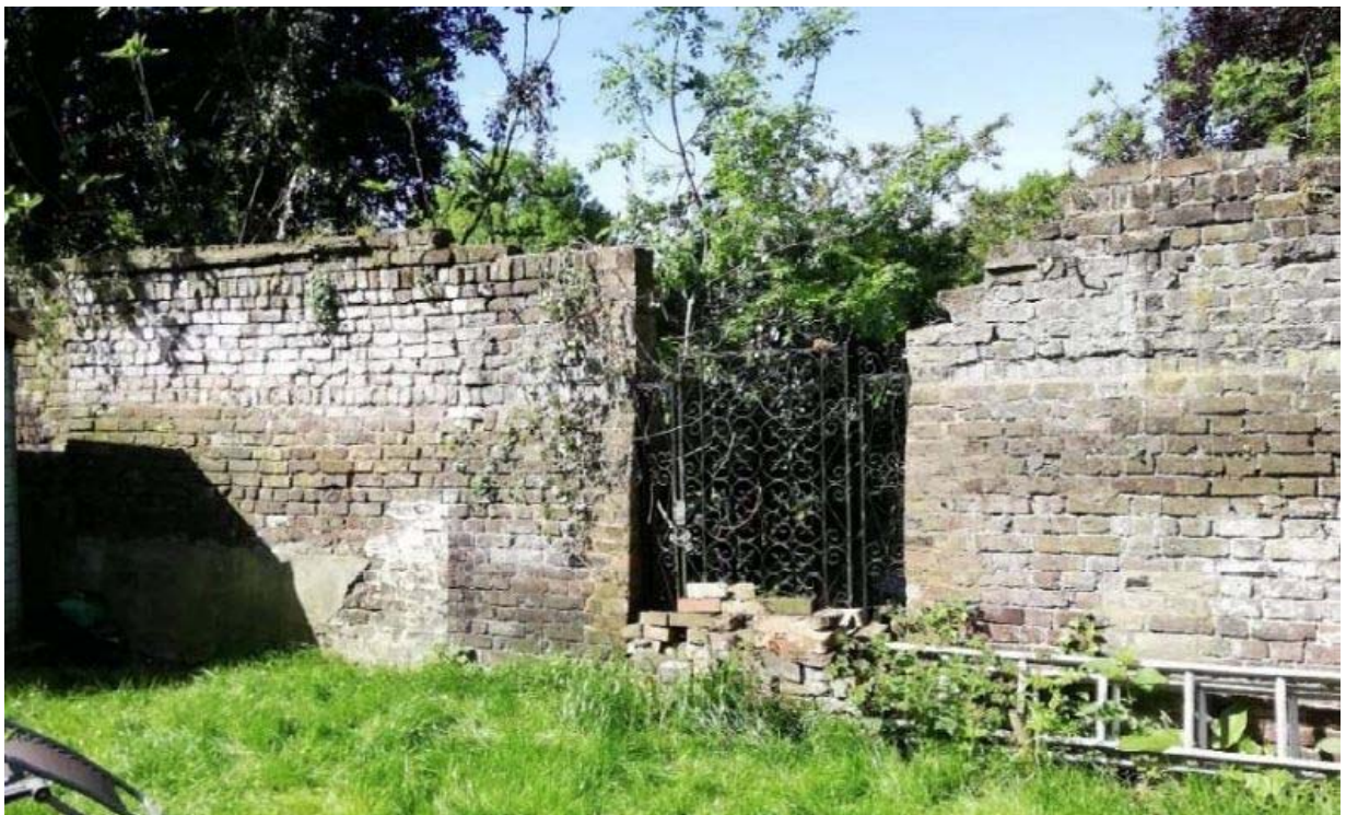
Photo 5: Boundary wall as viewed from No. 20 Perrin's Walk
