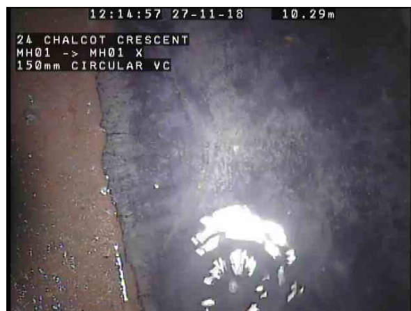
6, 00:02:09, 10.29m Finish node type, major connection without manhole, reference number: MH01 X / THAMES WATER SEWER
