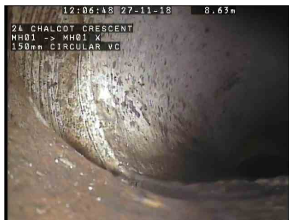
4, 00:01:32, 8.63m Joint displaced, medium
