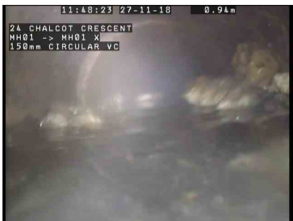
1, 00:00:18, 0.94m Settled deposits, coarse, 15% cross-sectional area loss, start
