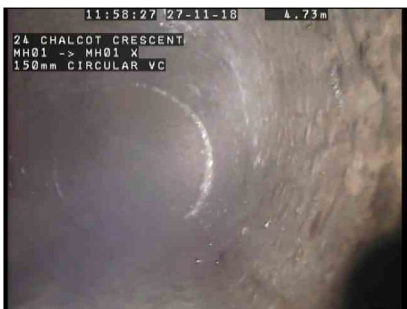
3, 00:00:51, 4.61m Settled deposits, other, 10% cross-sectional area loss, start / POSSIBLY GREASE
