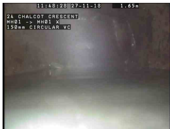
2, 00:00:24, 1.65m Connection other than junction at 02 o'clock, diameter: 100mm / UNKNOWN CONNECTION
