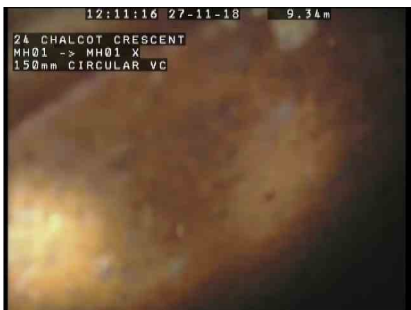
5, 00:01:40, 9.34m Joint displaced, medium
