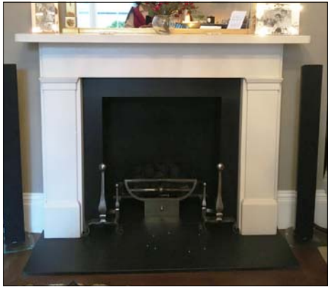
Photograph of existing Colebrook fireplace surround and Chesney's Morris Fire Basket from living room to be replicated within library. Refer to Chesney's drawings for details on fire basket.
