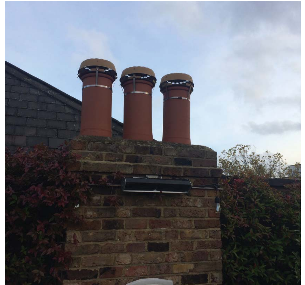
Roof Terrace Existing metal cowls to be replaced with Supply Bird cowls with peacemaker mat
