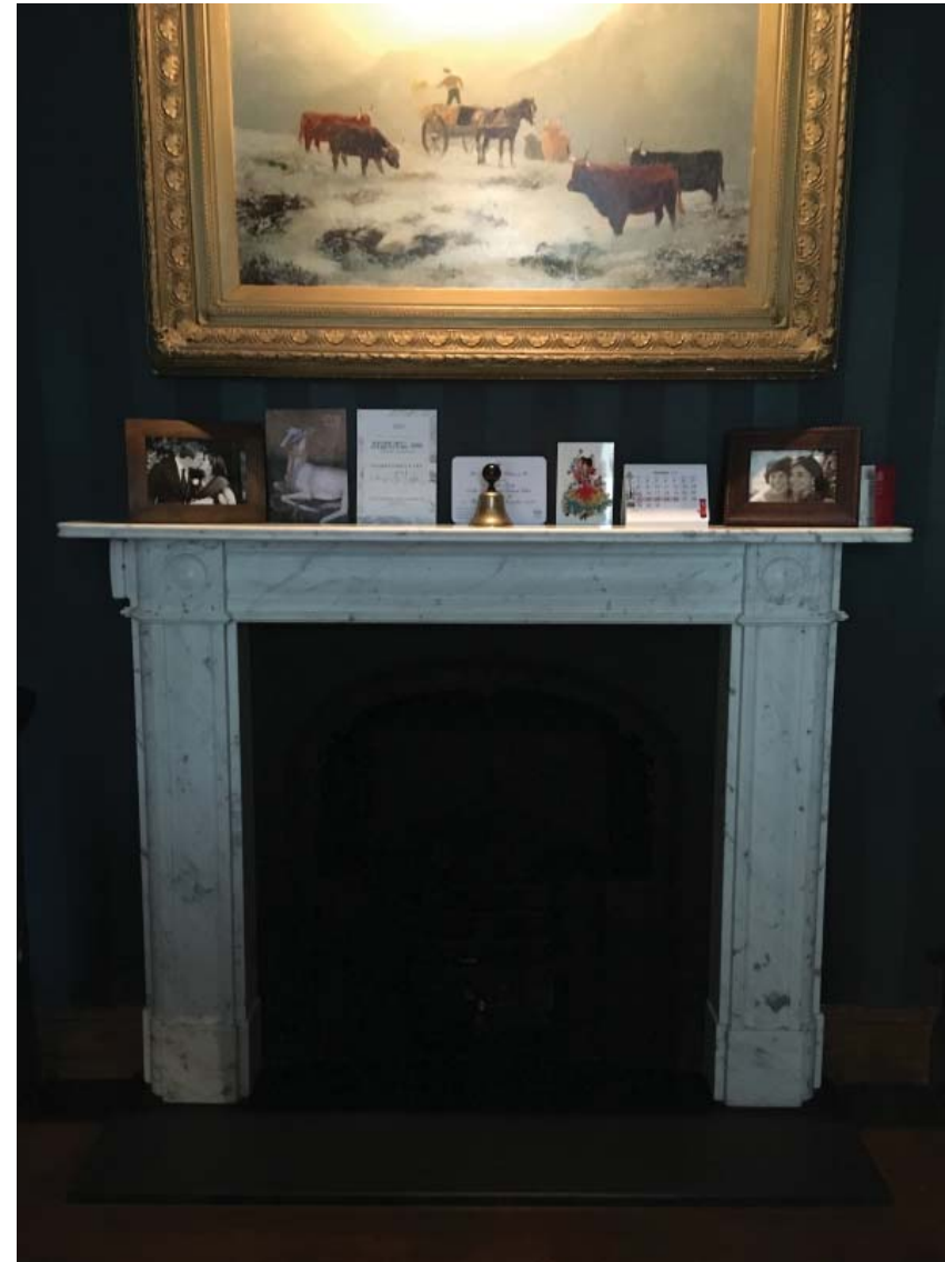
Ground Floor Library/Study Existing fireplace surround, inset and hearth to be removed
