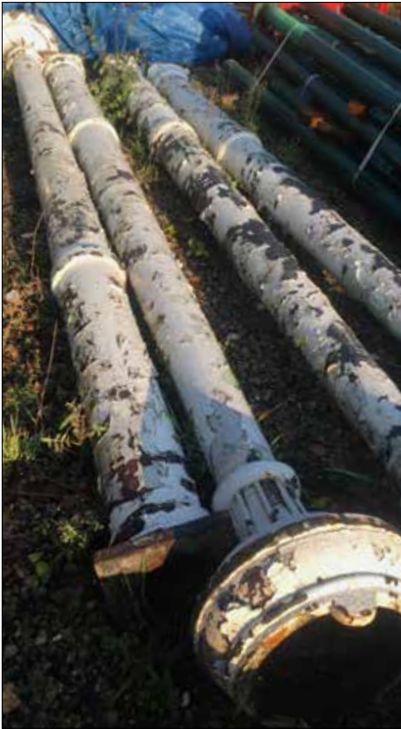
Cast iron columns (4 No.) - 4.5 metres high
