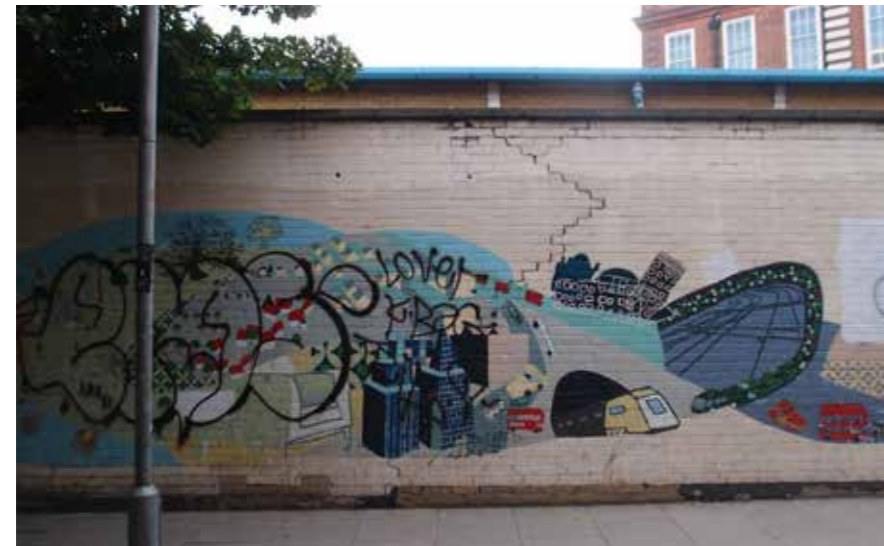
Existing external wall to North Gower Street
