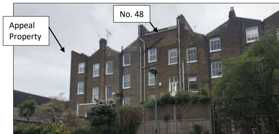
Rear Elevation of the Appeal Property and the Mansard Extension at No. 48
