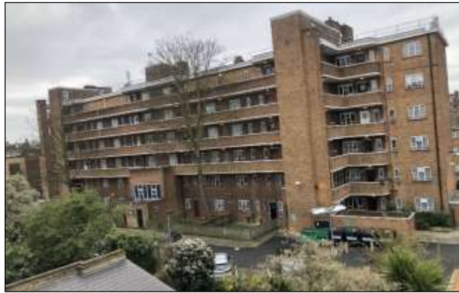
Flats to the Rear of the Appeal Terrace
