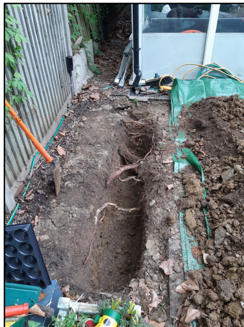
Photograph 2: Looking at 2m long trench (500mm deep) showing all roots uncovered during excavation.
