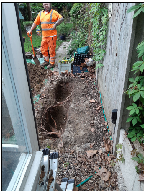
Photograph 3: Looking south along the excavated trench.
