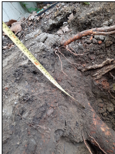
Photograph 6: Showing the depth of the largest root at 300mm below ground level.
