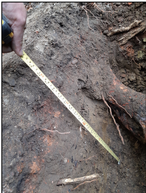
Photograph 5: Showing the depth of the trench, 500mm or greater than 500mm.
