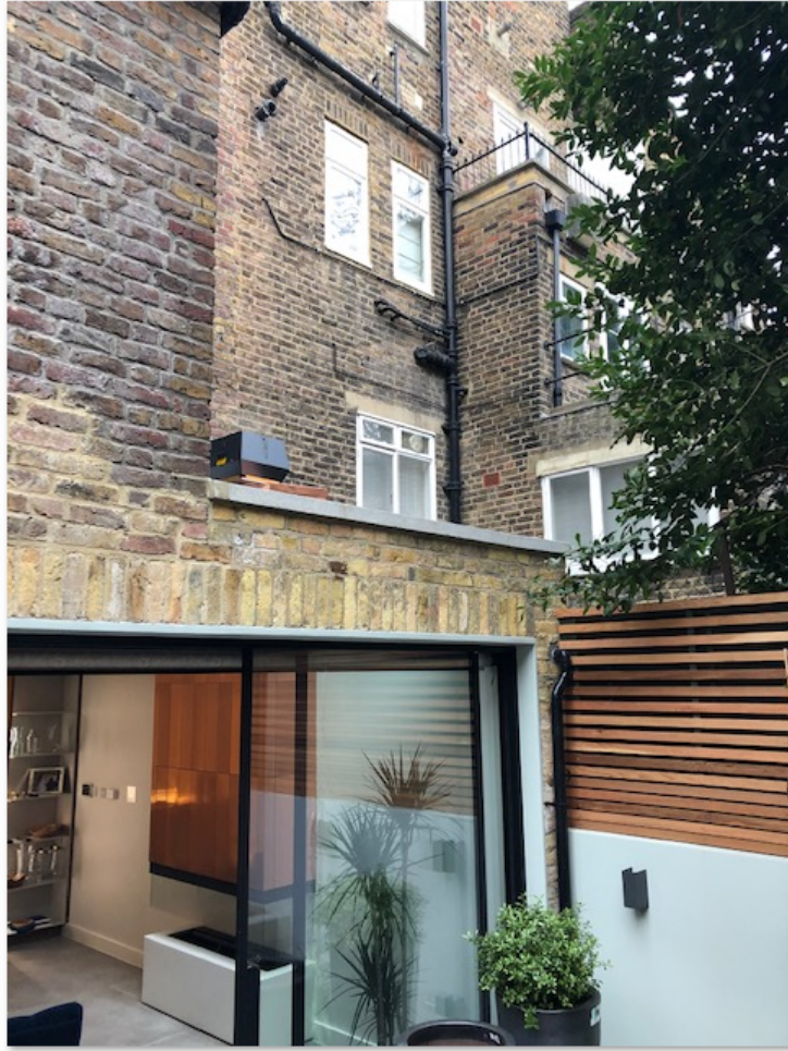
Photo 1 showing rear extension as built and boundary wall with no.16
