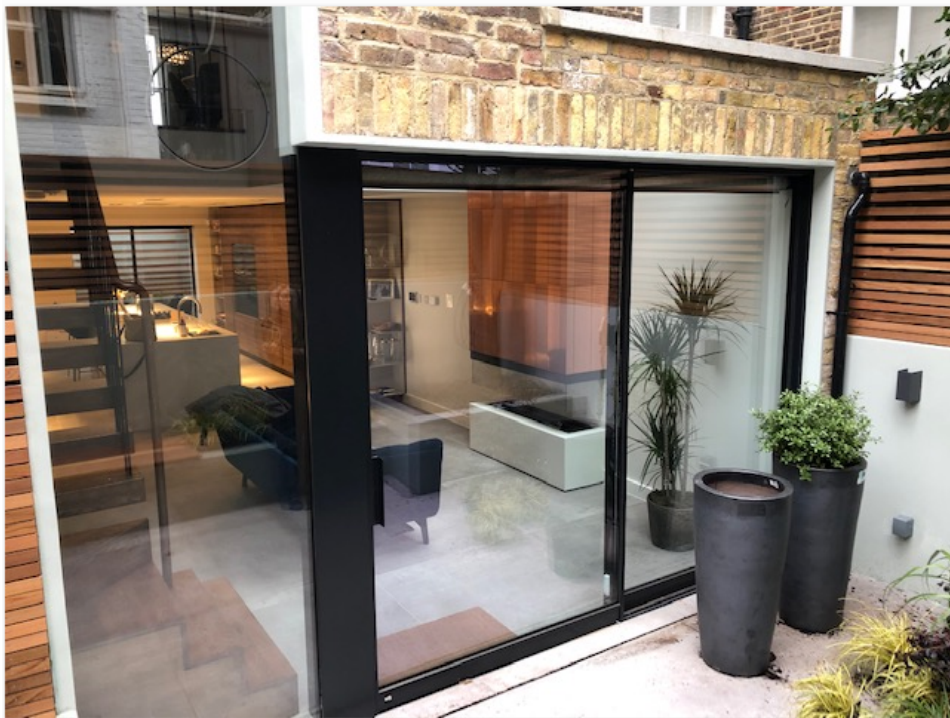
Photo 2 showing rear extension fenestration and join with existing closet wing.
