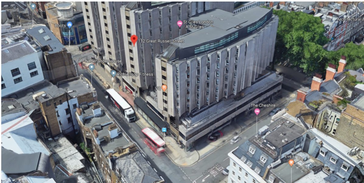
1) Birds eye view of Great Russell Street and Adeline Place Elevations (vehicular entrance on to Adeline Place).
