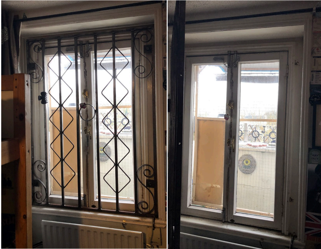
Figure 7: Internal view of left hand side window at third floor bedroom (to the left with security grilles closed, to the right with security grilles open (Flat C)
