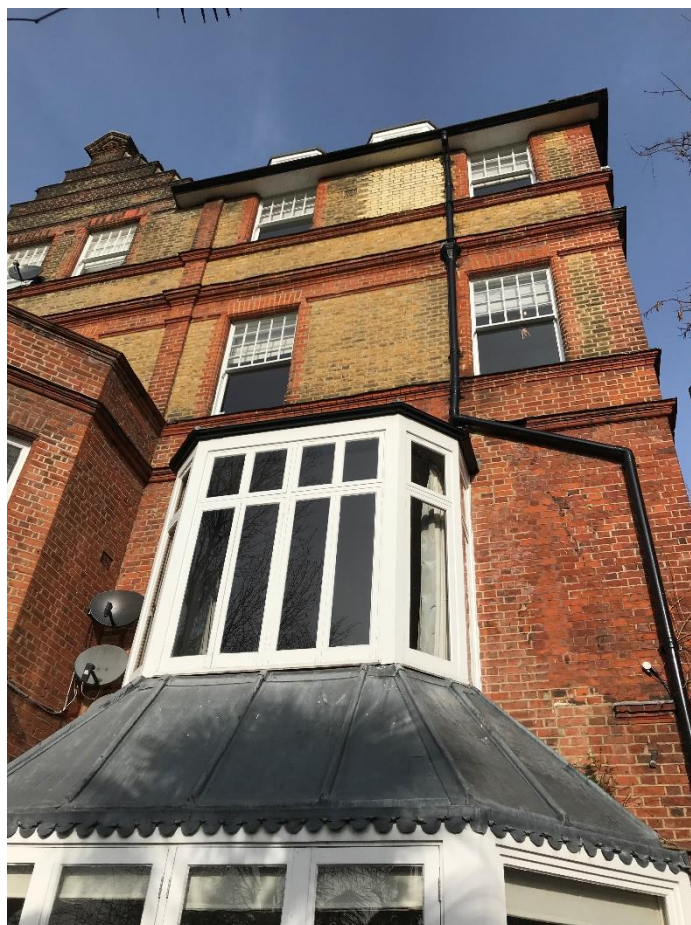
Plate 6: Rear Elevation showing brickwork disturbance around bay window and cut off of brick banding
