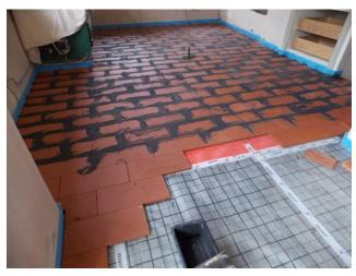
The Jupiter Screed Replacement Tile was used to provide the ideal substrate for the large-format finished floor tiles. The SRT system decouples the finished floor and allows Jupiter to guarantee finished floor tiles against failure for five years.
