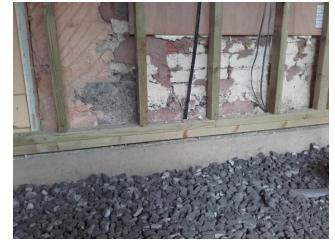
As an alternative to a conventional slab TechnoPor Glass Foam was used. Adopting this method of construction forms a strong and insulated base without the drying out time of a concrete slab.
