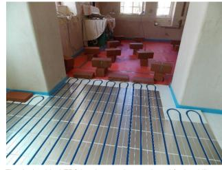
The Jupiter Ideal EPS heating panel was selected for its ability to deliver superb heat output rapidly and, equally importantly, evenly to prevent cold spots on the floor.
