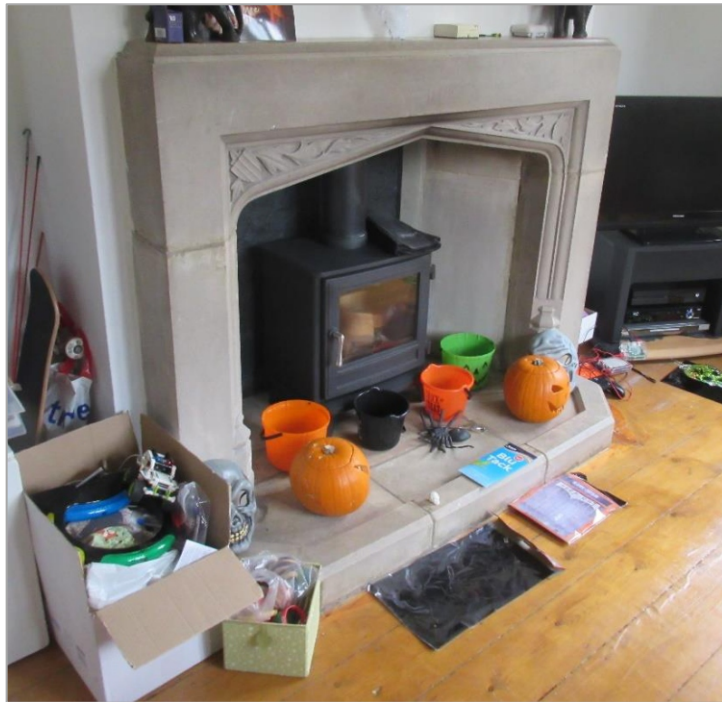
Figure 4: The sitting room has a boarded floor and a C20 Tudor-style stone fireplace
