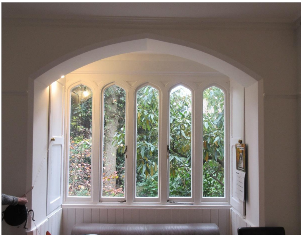
Figure 5: Dining room bay window within pointed and chamfered arched recess
