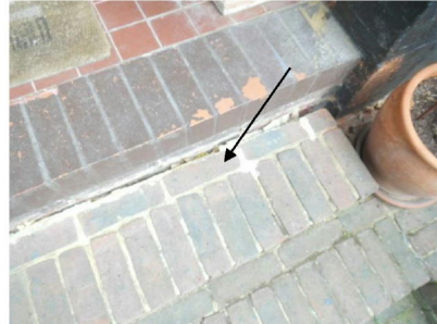
Cracks to front steps
