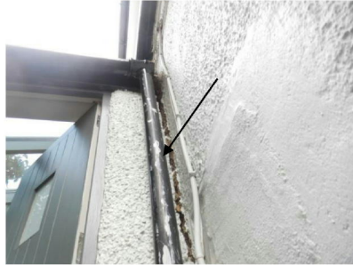
Front - vertical separation crack at junction of single storey structure and main building
