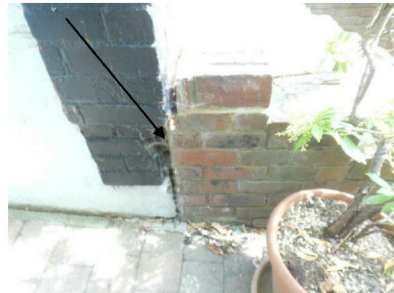
Separation crack to front steps
