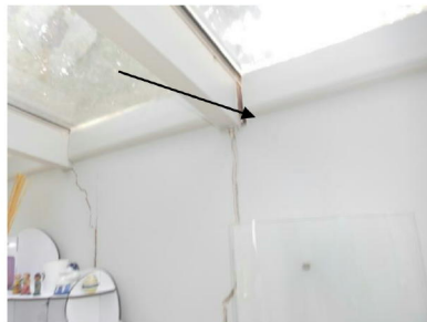
Study – vertical crack and separation of the roof structure
