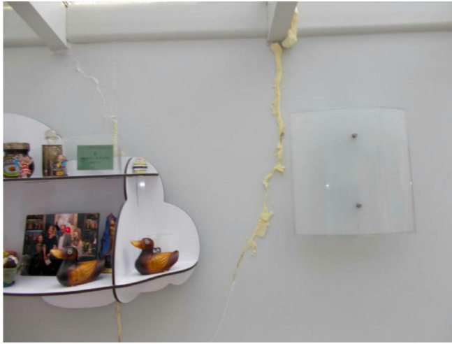
View of cracking to internal walls on left hand side of property
