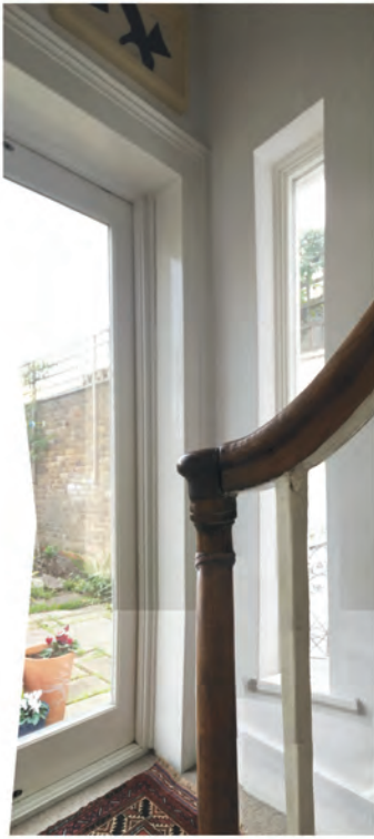
Fig. 18 - Modern door and window in ground floor hallway
