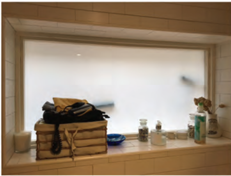
Fig. 20 - Internal window in basement shower room
