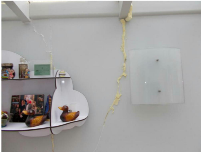
View of cracking to internal walls on left hand side of property
