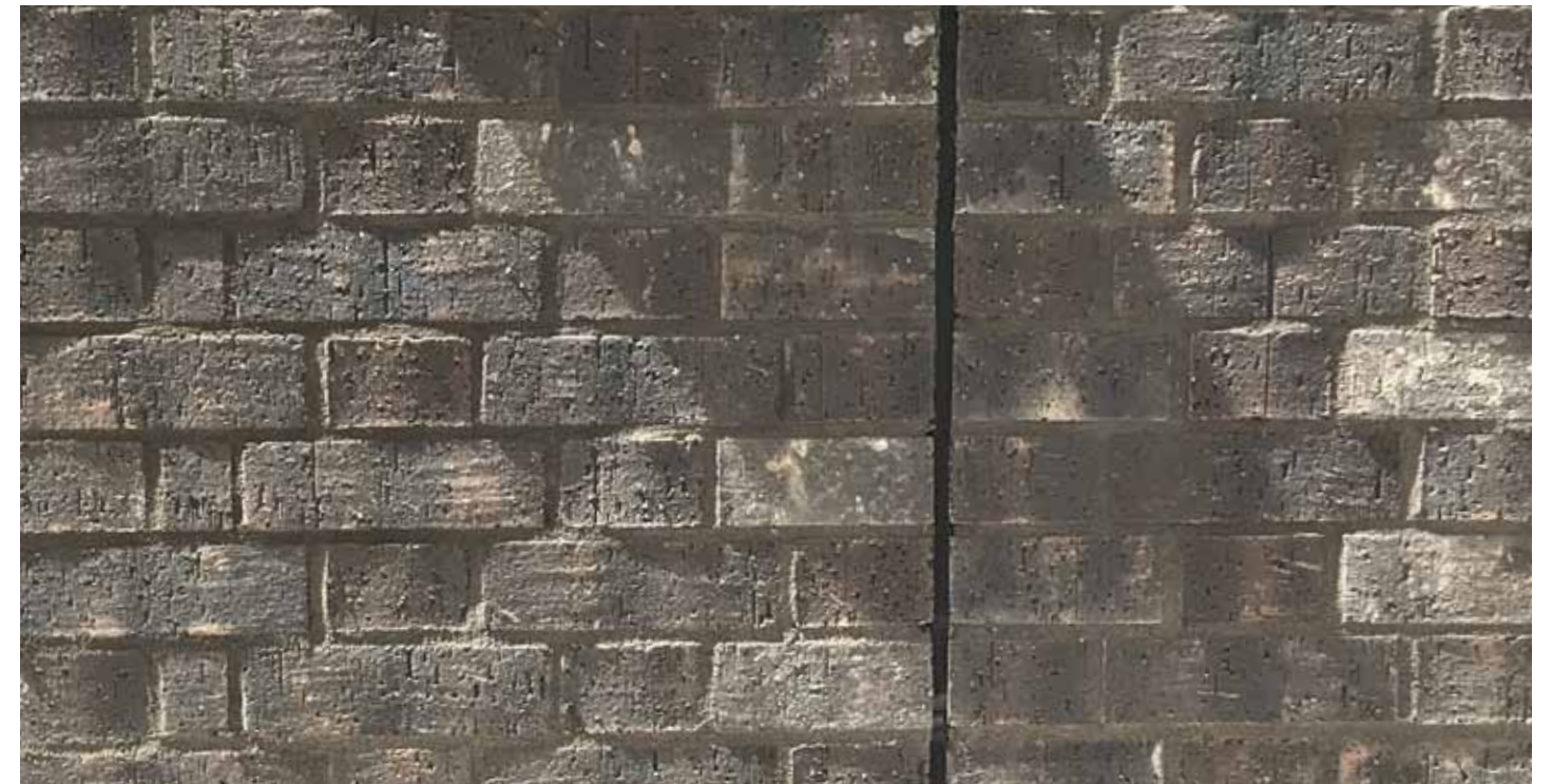
Brick sample panel
