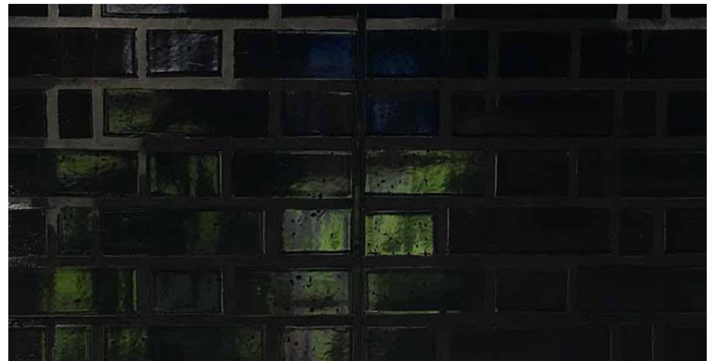
Brick sample panel
