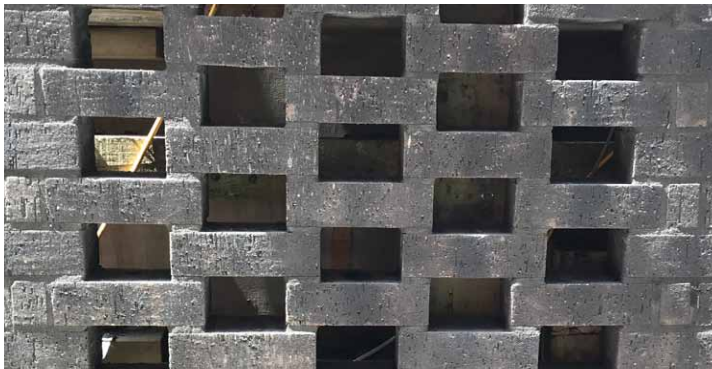
Brick sample panel
