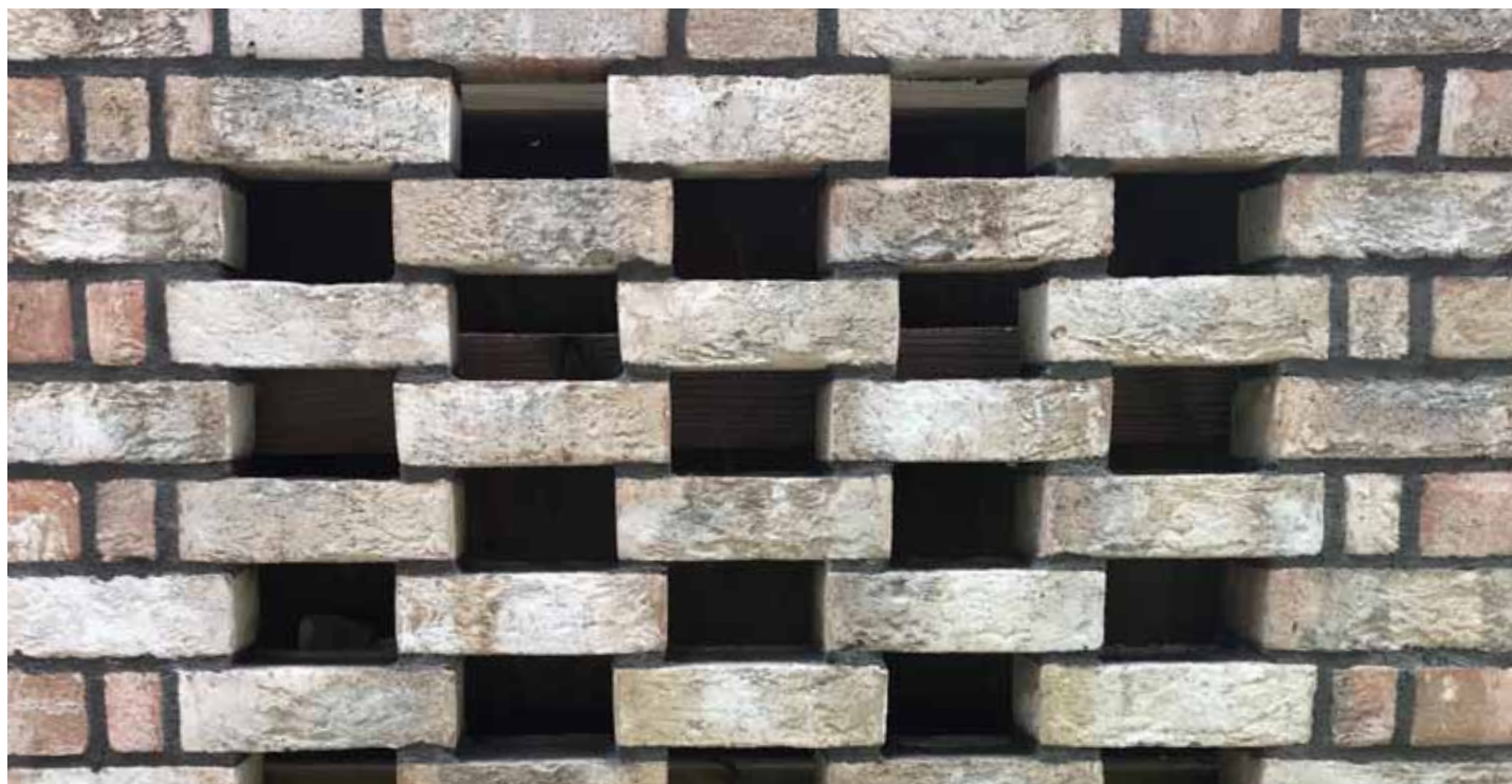
Brick sample panel
