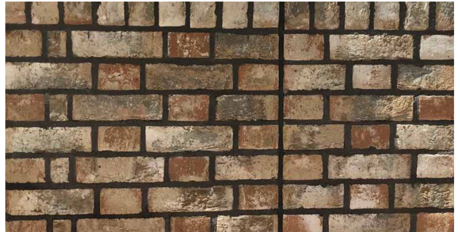
Brick sample panel
