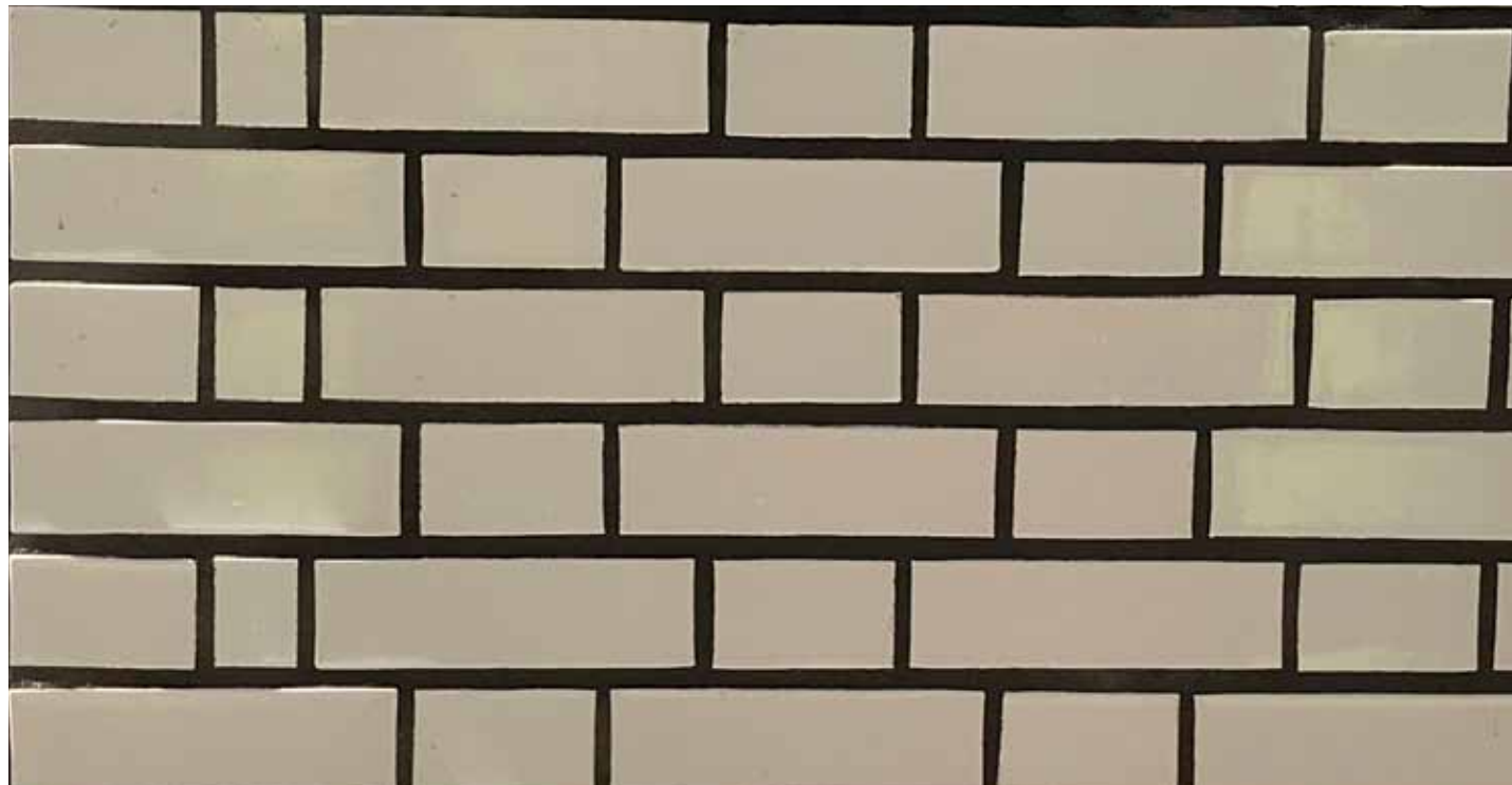
Brick sample panel
