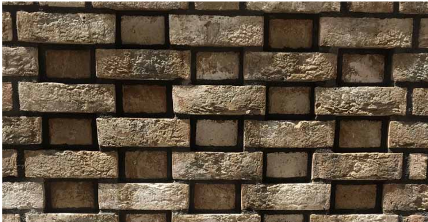
Brick sample panel
