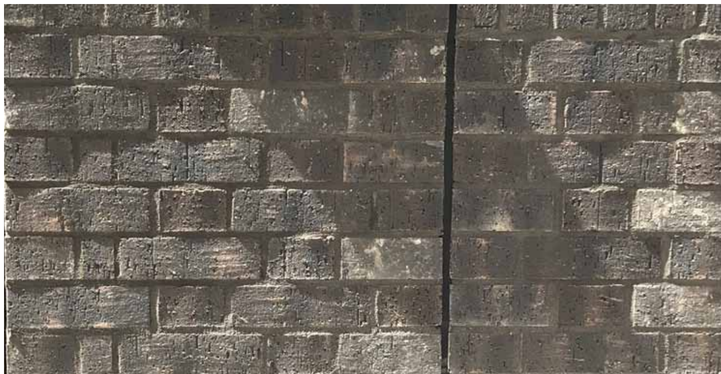
Brick sample panel
