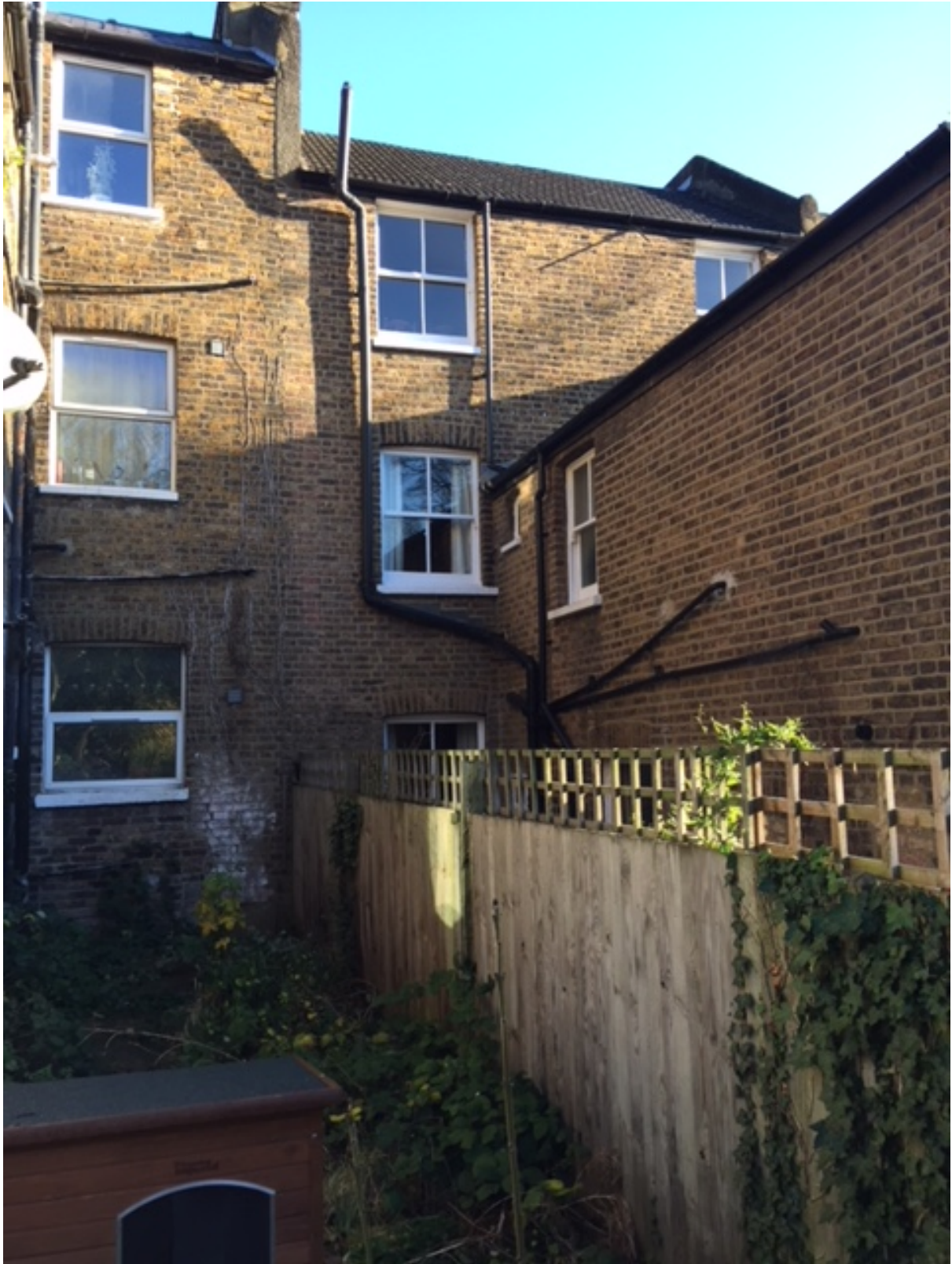
Existing rear elevation of application property and no. 6
