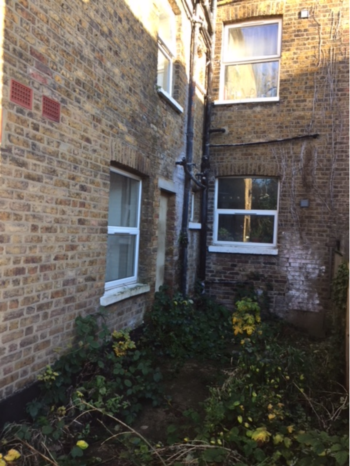
Existing ground floor rear elevation of application site
