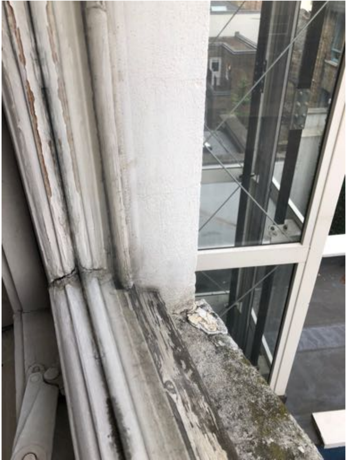
Fig 2: Evidence of existing sash box as seen on Second Floor (External)
