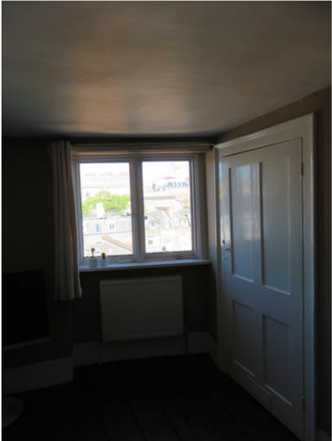
Fig 5: Existing Third Floor Window to curved wall (Bedroom)
