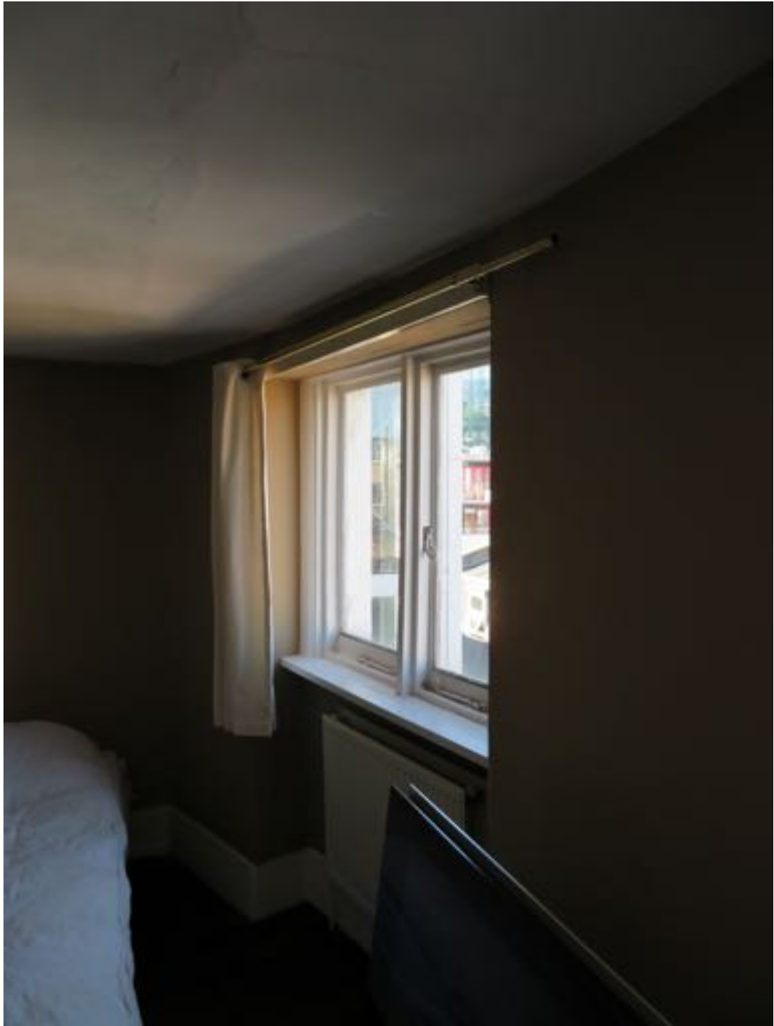
Fig 4: Existing Third Floor Window to curved wall (Bedroom)
