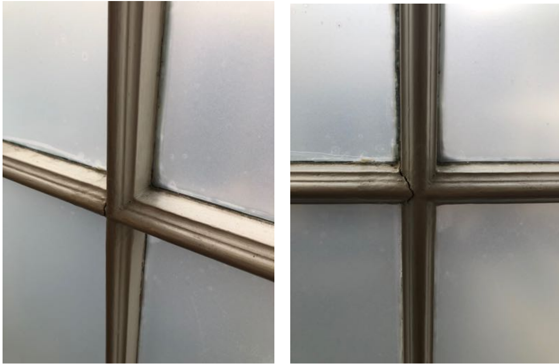
Fig 6 & 7: Glazing bar to First Floor rear room
