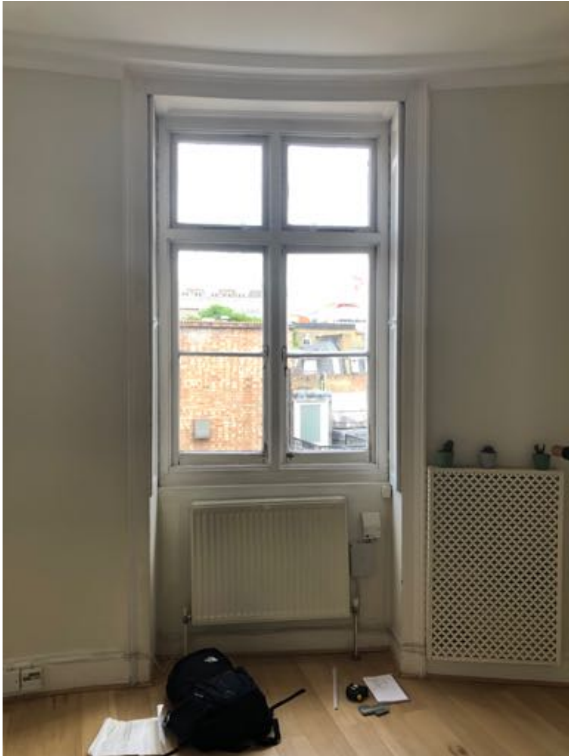
Fig 1: Second Floor Window – RHS as Viewed Internally
