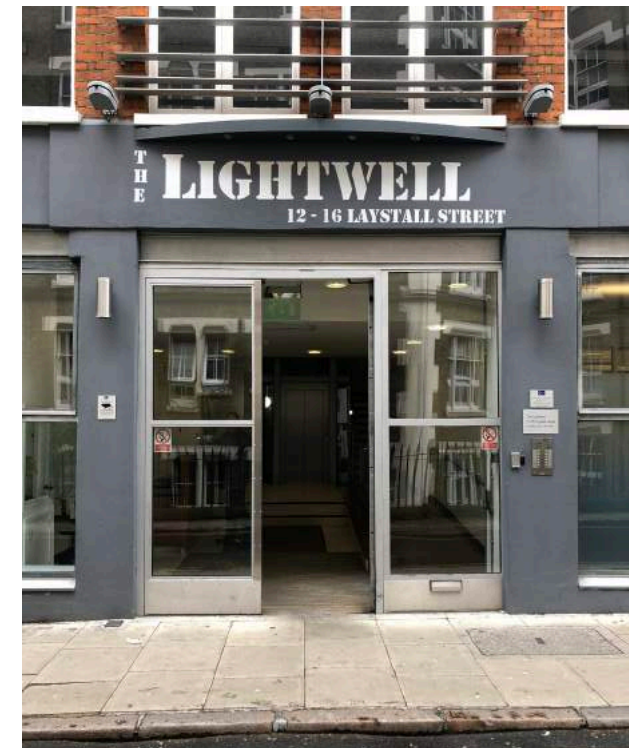
Uninviting entrance and off centered entry doors
