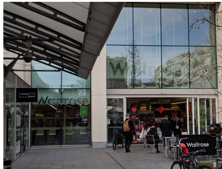
Current signage in-situ/Proposed signage location
