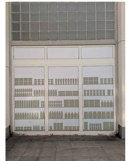
Current signage in-situ/Proposed signage location
