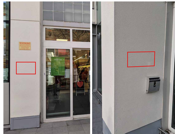
Current signage in-situ/Proposed signage location
