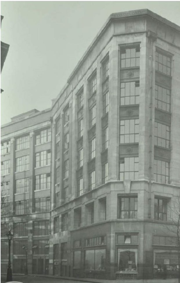
Figure 2: 1915 photograph of Kodak House showing original appearance and arrangement.
