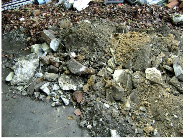
Concrete and rubble dug out of test pits 1, 2 and 3.
