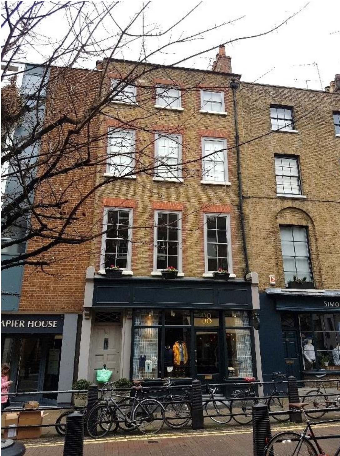
Figure 1. Front elevation of the Site, comprising four storeys plus basement.
