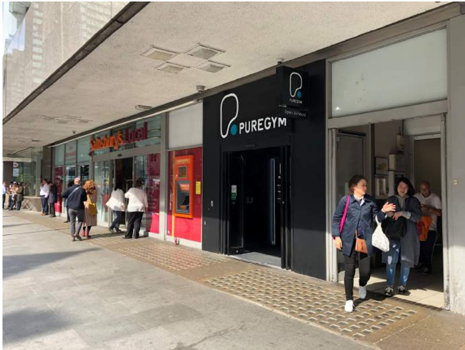
Existing shop front, entrance left, exit right
