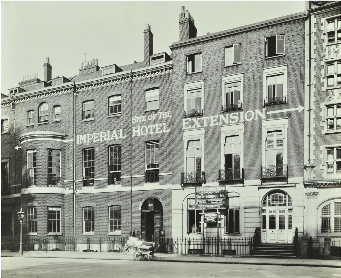
Fig 12 (left). Part of Bolton House and Sir Thomas Lawrence’s House earmarked for demolition in 1910, the first phase of the first Imperial Hotel just visible on the right of the image (LMA).
