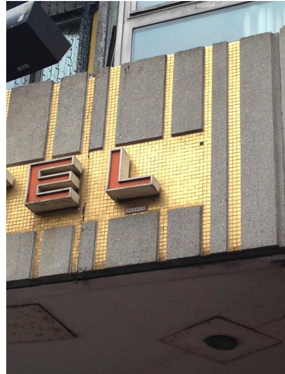
Fig 20 (left). Detail of stained concrete and mosaic before cleaning. Fig 21. The same area after trial cleaning
