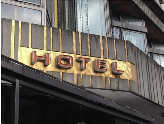
Fig 17 (left). Detail of textured concrete cladding with gold mosaic and original 1960s signage Fig 18 (right). The ground-floor projection on the front wing
