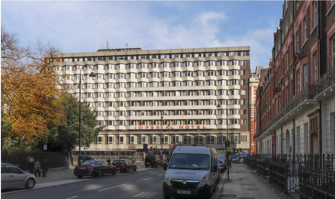
Fig 1. The Imperial Hotel, Russell Square: front elevation viewed from the west
