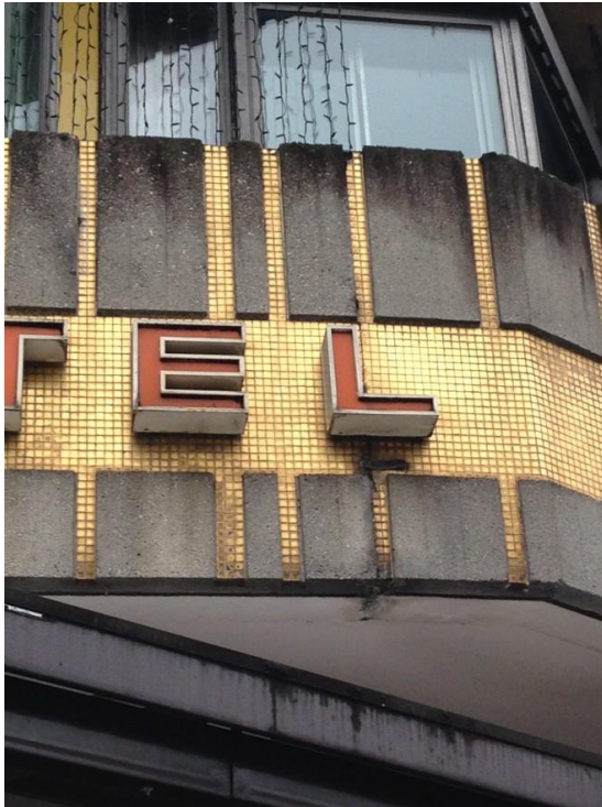
Fig 20 (left). Detail of stained concrete and mosaic before cleaning. Fig 21. The same area after trial cleaning
