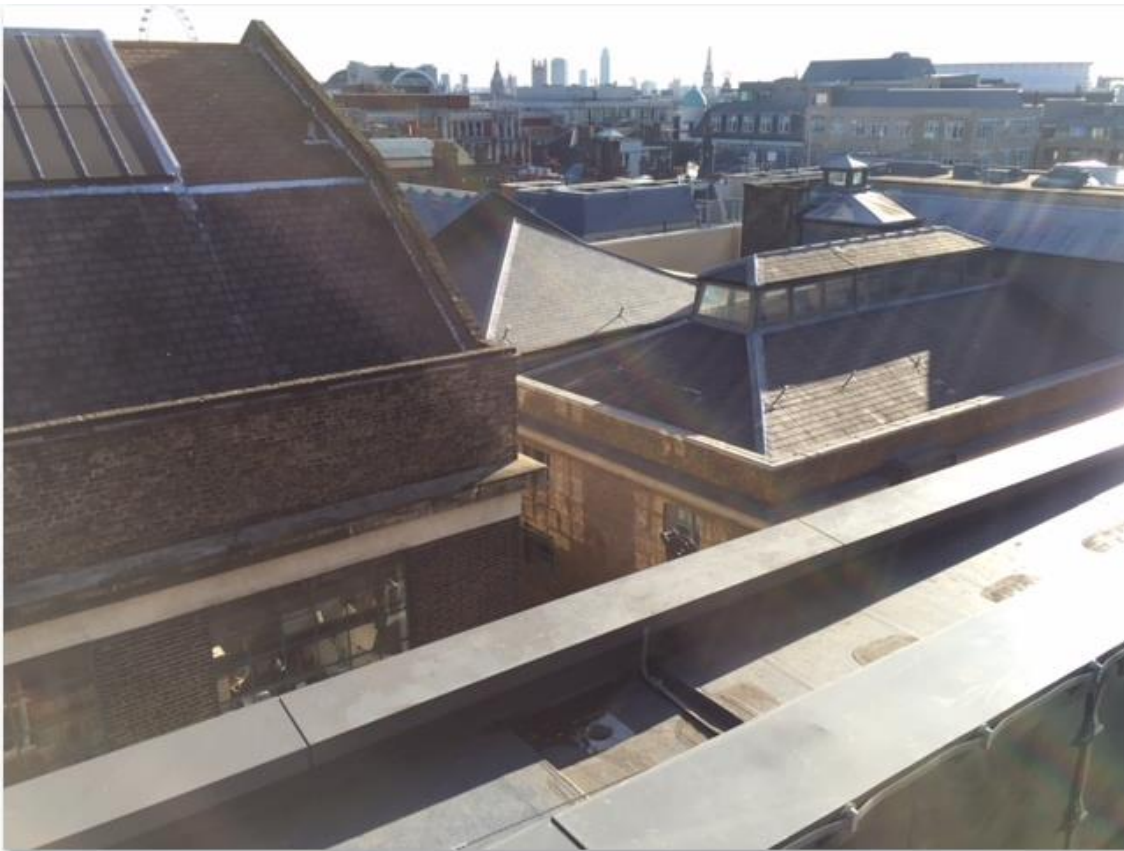
Photo 2: View south from the roof terrace
