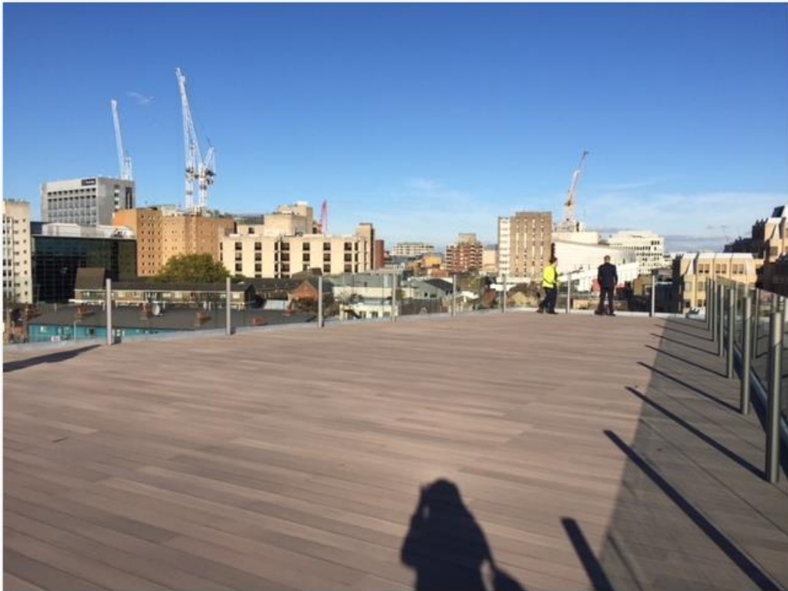
Photo 4: Roof terrace area
