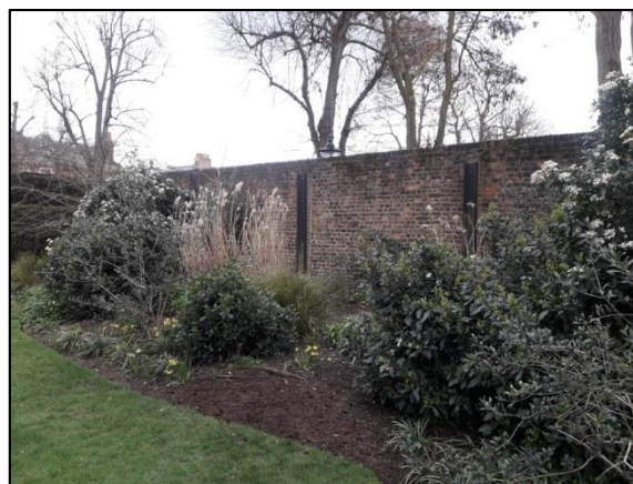
Photo 3: Steel supports securing the boundary wall
