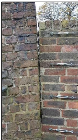
Photo 4: Open joint between pier and wall
