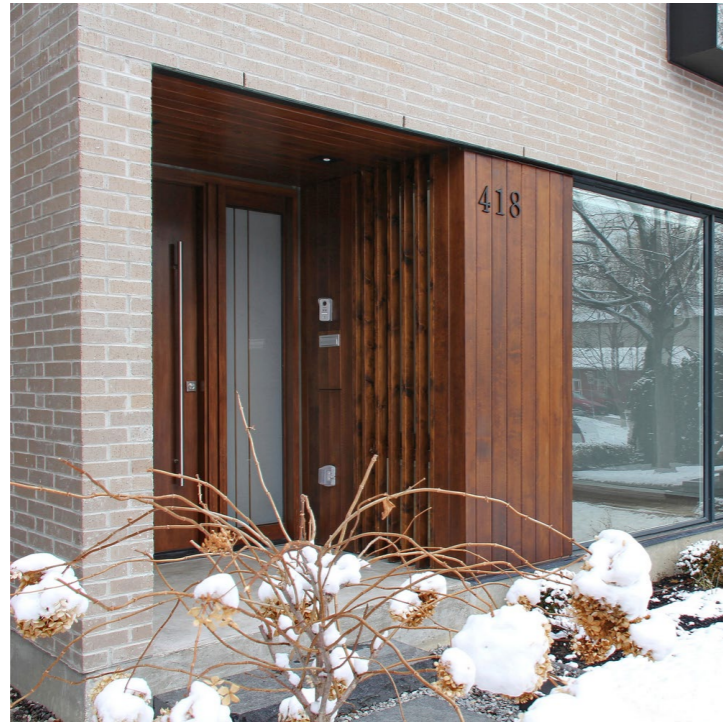
1. Timber to entrance
