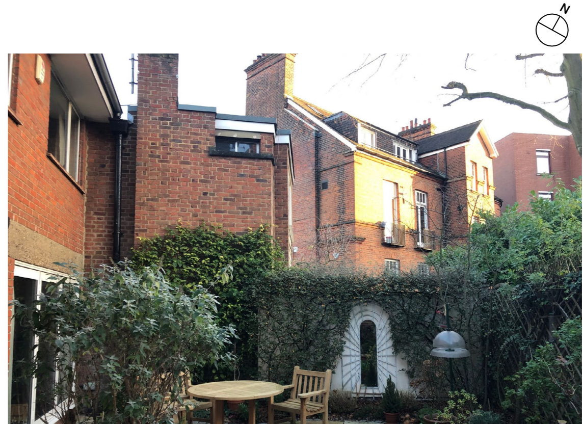
Existing boundary condition between 4a & 4b
