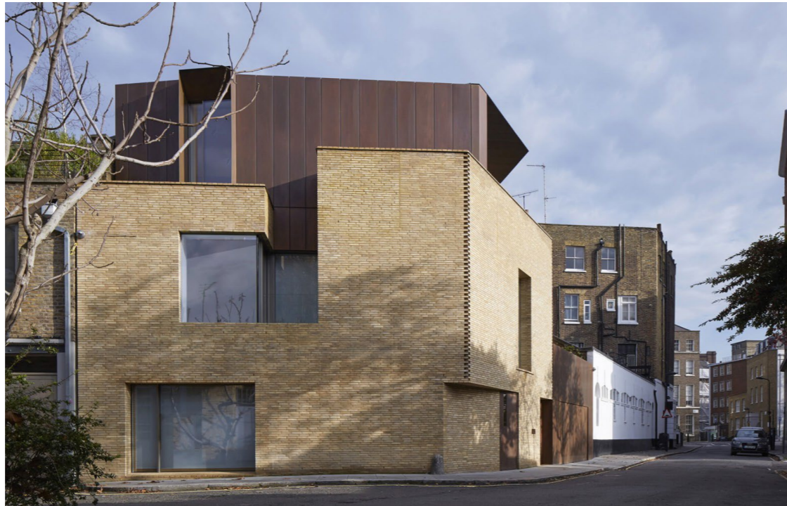
Roof intersecting a carved brick form. Bloomsbury Conservation Area, London. RIBA National Award 2015. Jamie Fobert Architects
