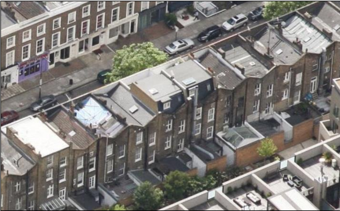
Photo 2 – aerial photograph showing rear of Boundary Road with differing roof patterns.
