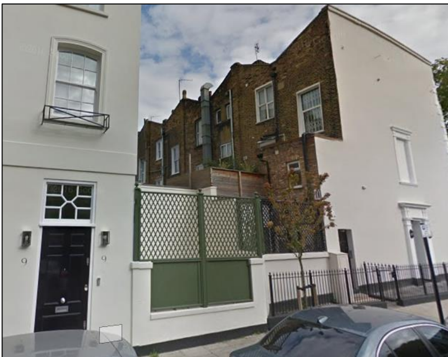
Photo 1 - First floor rear extension at 132 Boundary Road
