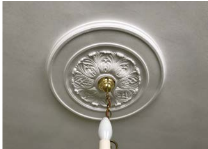
Ceiling Rose (non-original)
