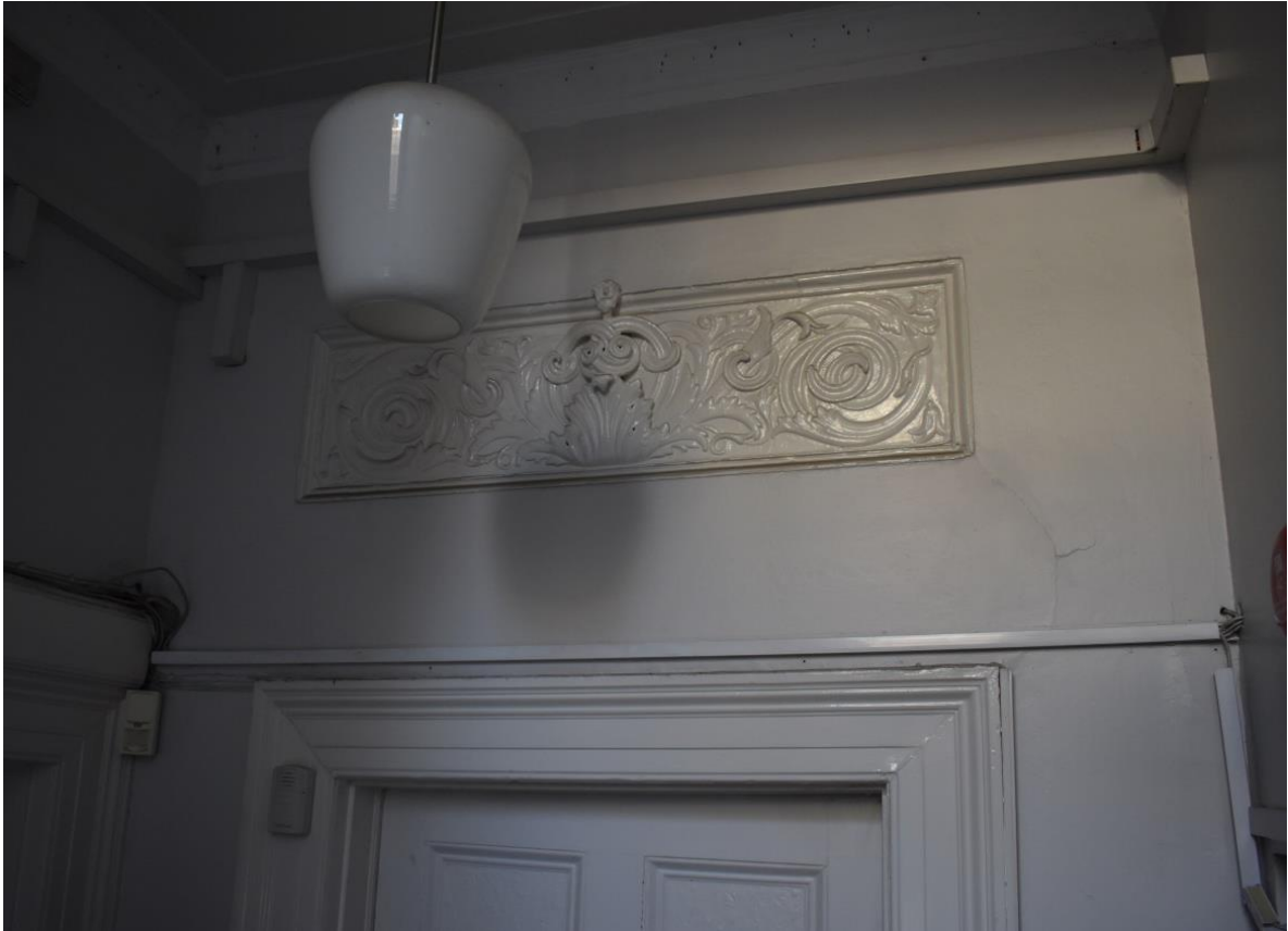
Fig 14 Original door surround and plasterwork above entrance to first floor front room of No.38
