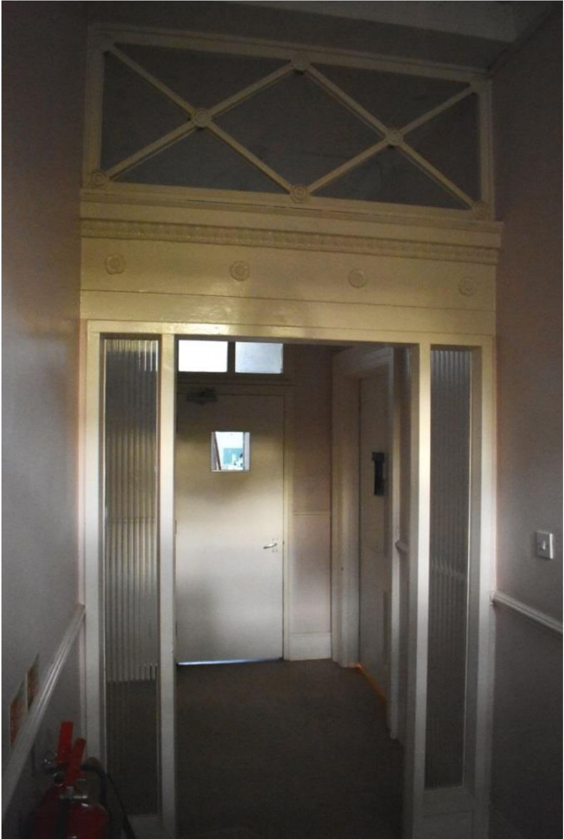
Fig 13 Inner doorway of No.38 Gordon Square, a combination of original (upper) and 20th-century (lower) joinery
