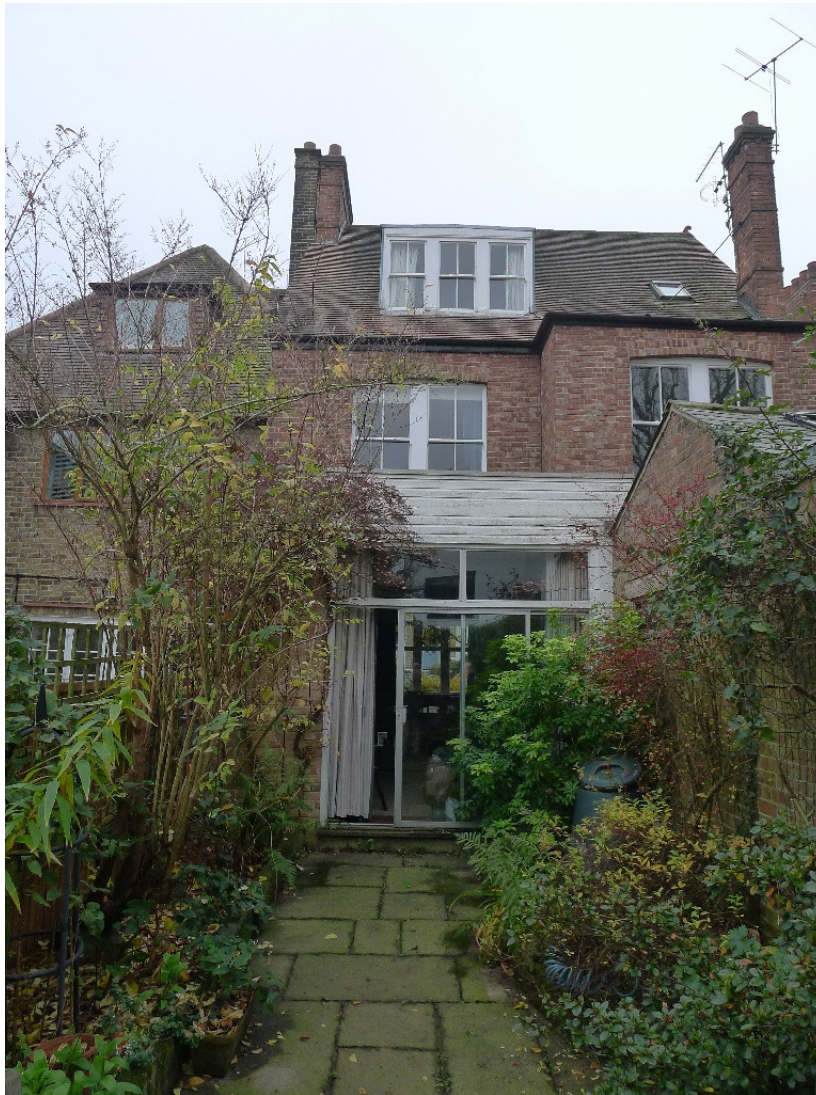
General view of rear elevation
