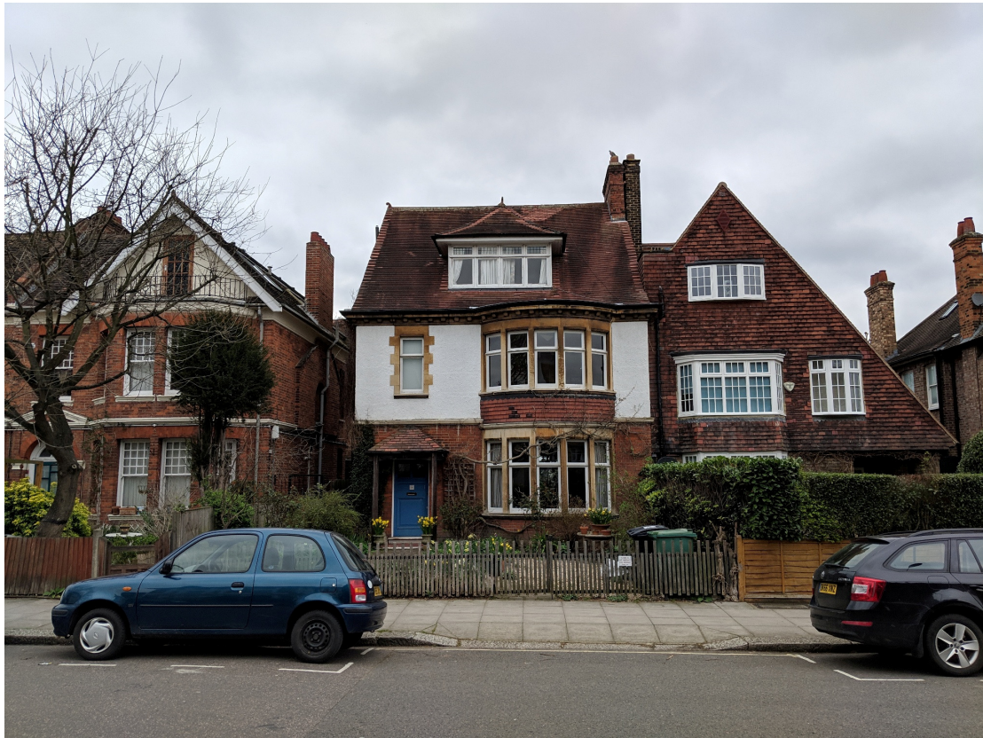
General view from St Albans Road
