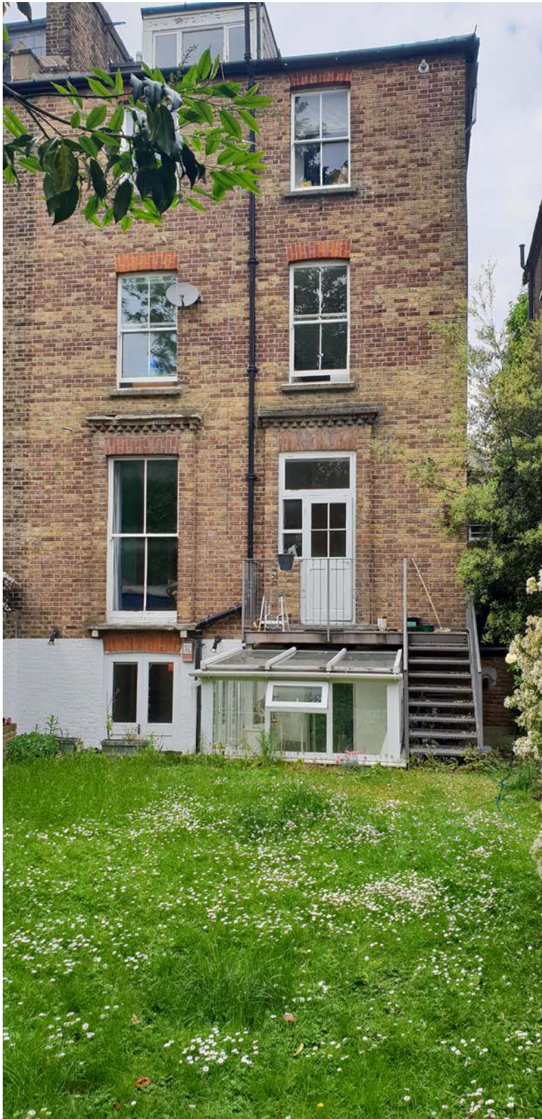
15 Lyndhurst Road- Rear elevation
