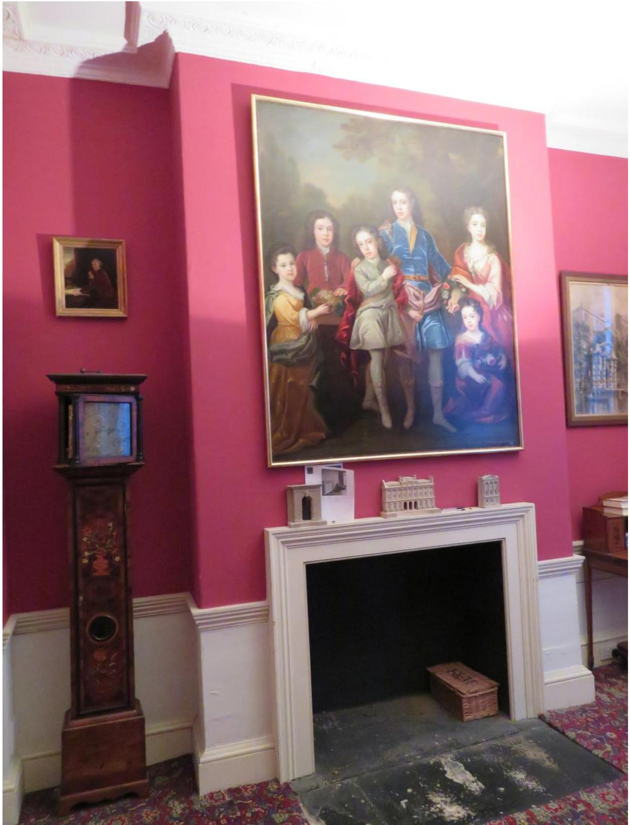
Fig. 2 – Existing timber fireplace surround, 6 Fitzroy Sq ground floor rear room, to be removed.
