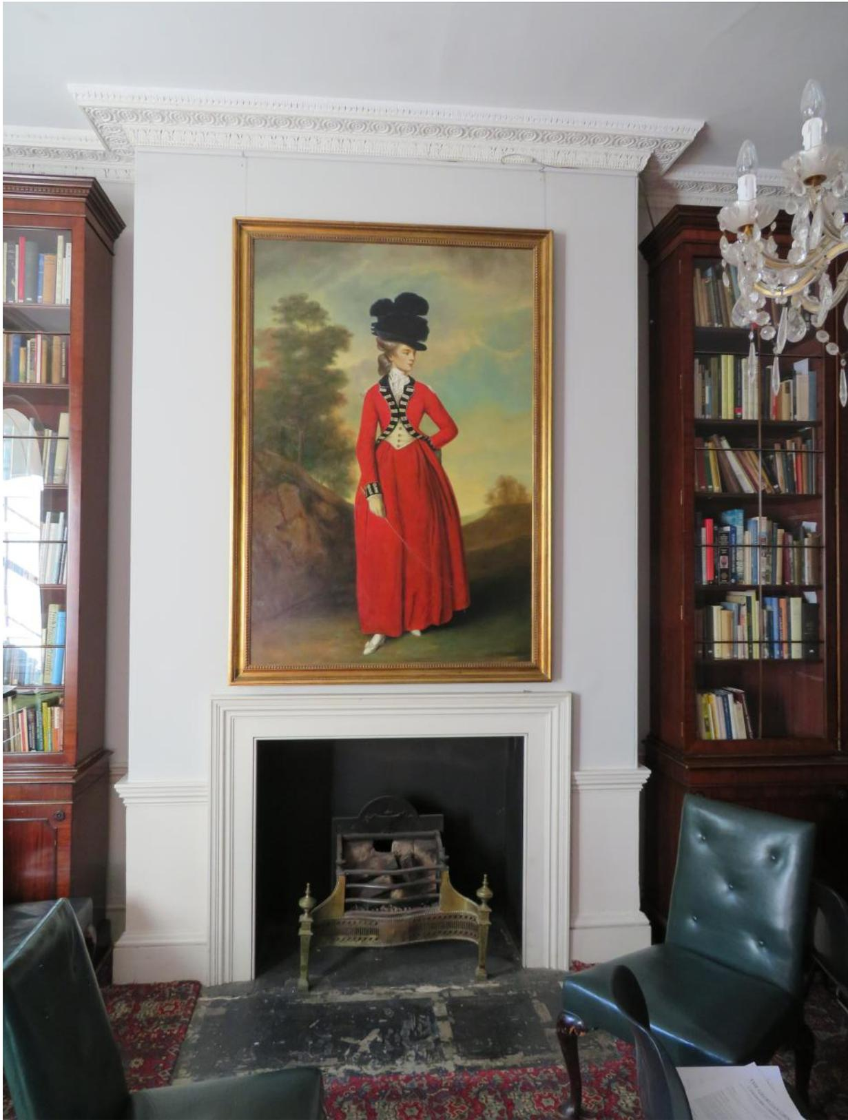
Fig. 1 – Existing timber fireplace surround, 6 Fitzroy Sq ground floor front room, to be removed.
