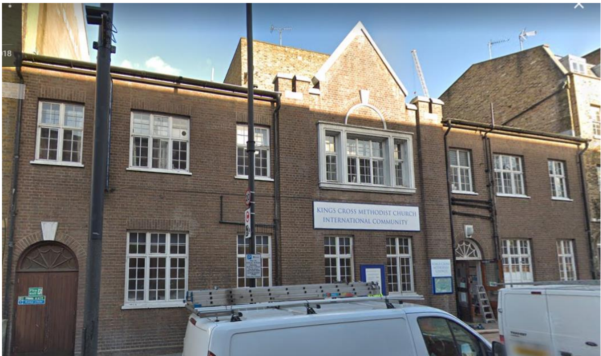
4. Crestfield Street façade
