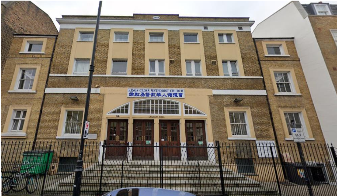
1. Birkenhead Street façade (positive contributor)
