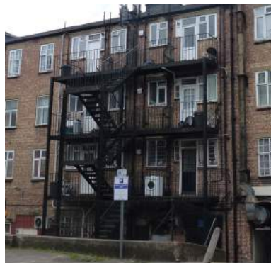
Retaining Existing Stairs
