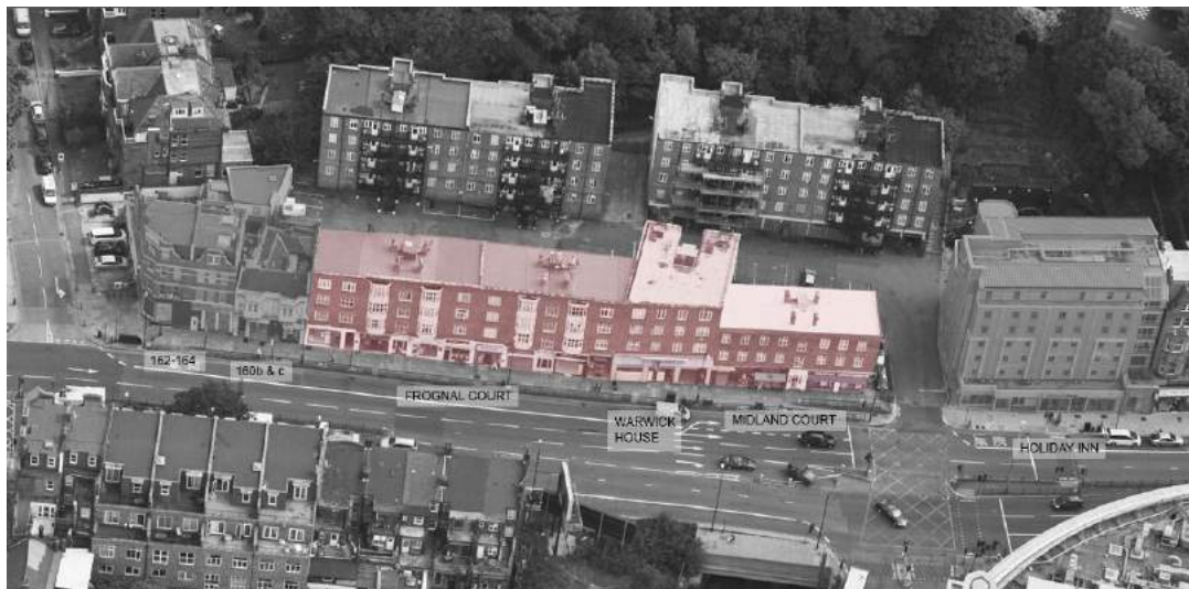
Aerial view of the Frognal Court Estate. Red denotes the area for development.
