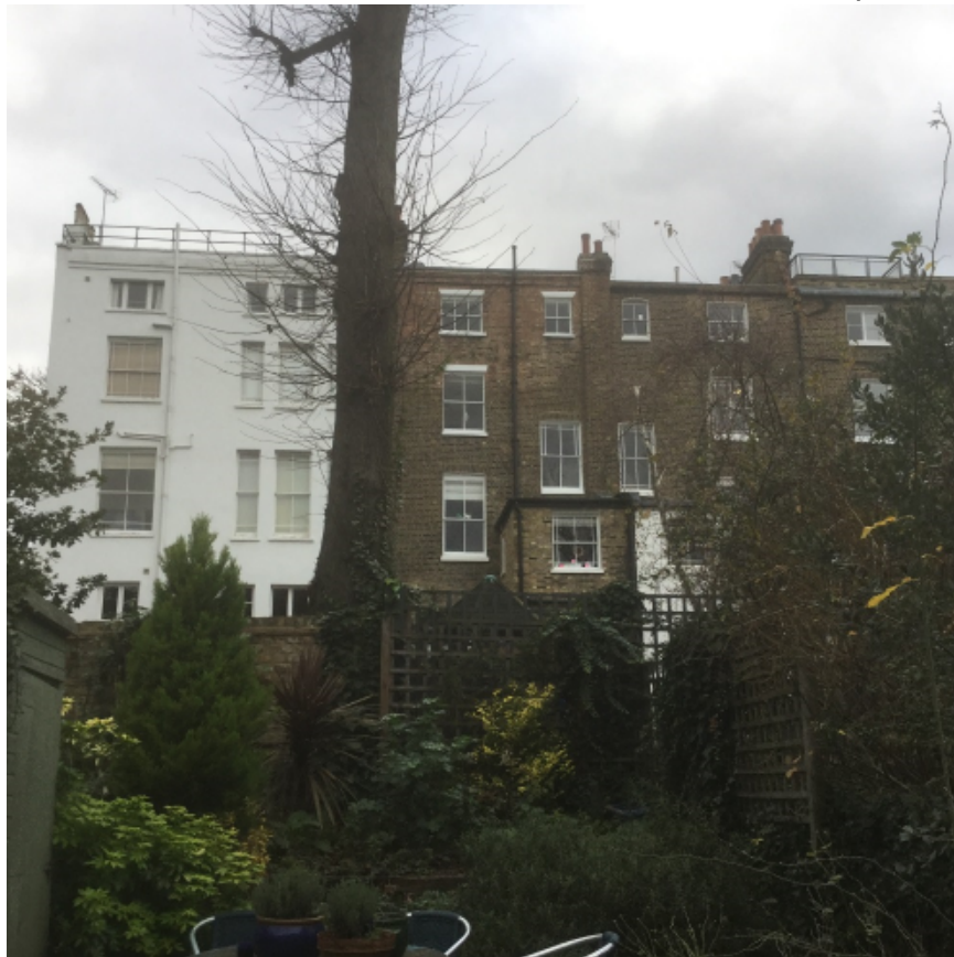
8. View towards the rear garden of the application site.
