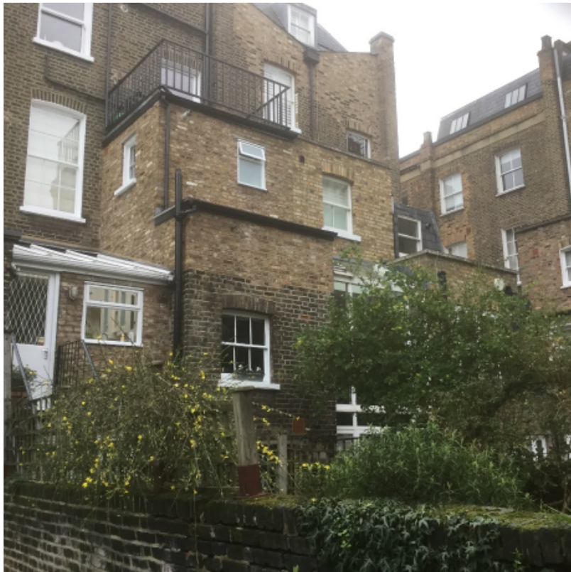
6. View towards nos. 22 and 24 Fitzroy Road. Note trellis and elevated staircase to the ground floor level.
