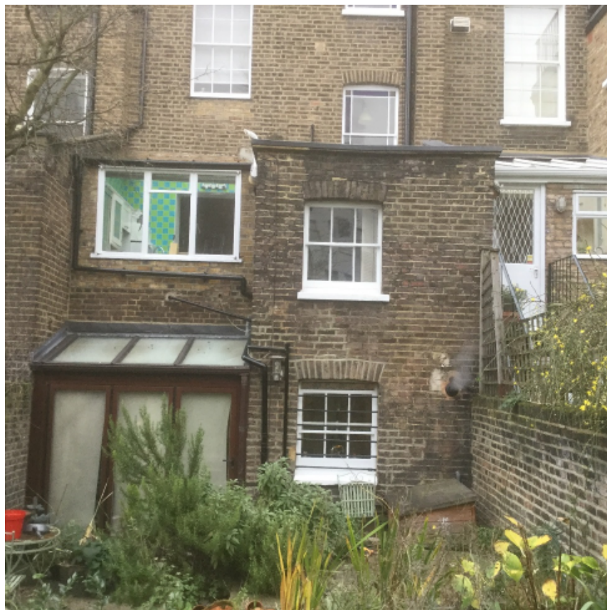
4. Rear elevation of the application site.
