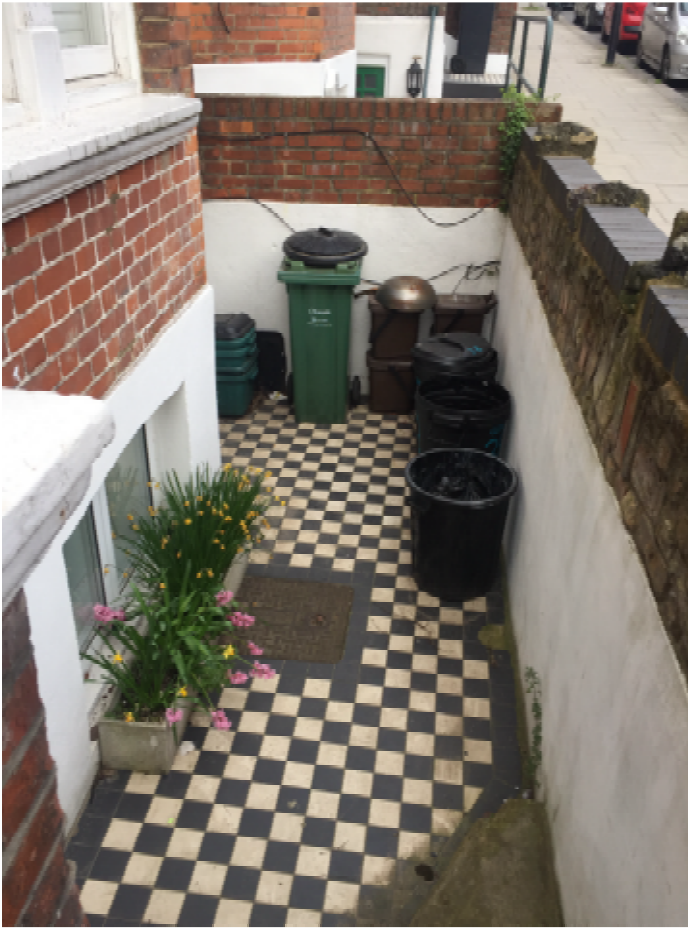
Photo 6 – Front lightwell to be deepened
