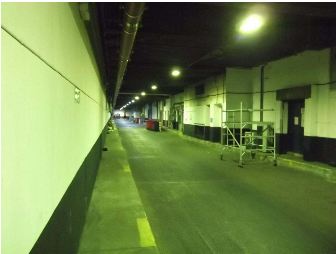
Figure 10: View looking north along service road. Note: items of mechanical plant at other sites
