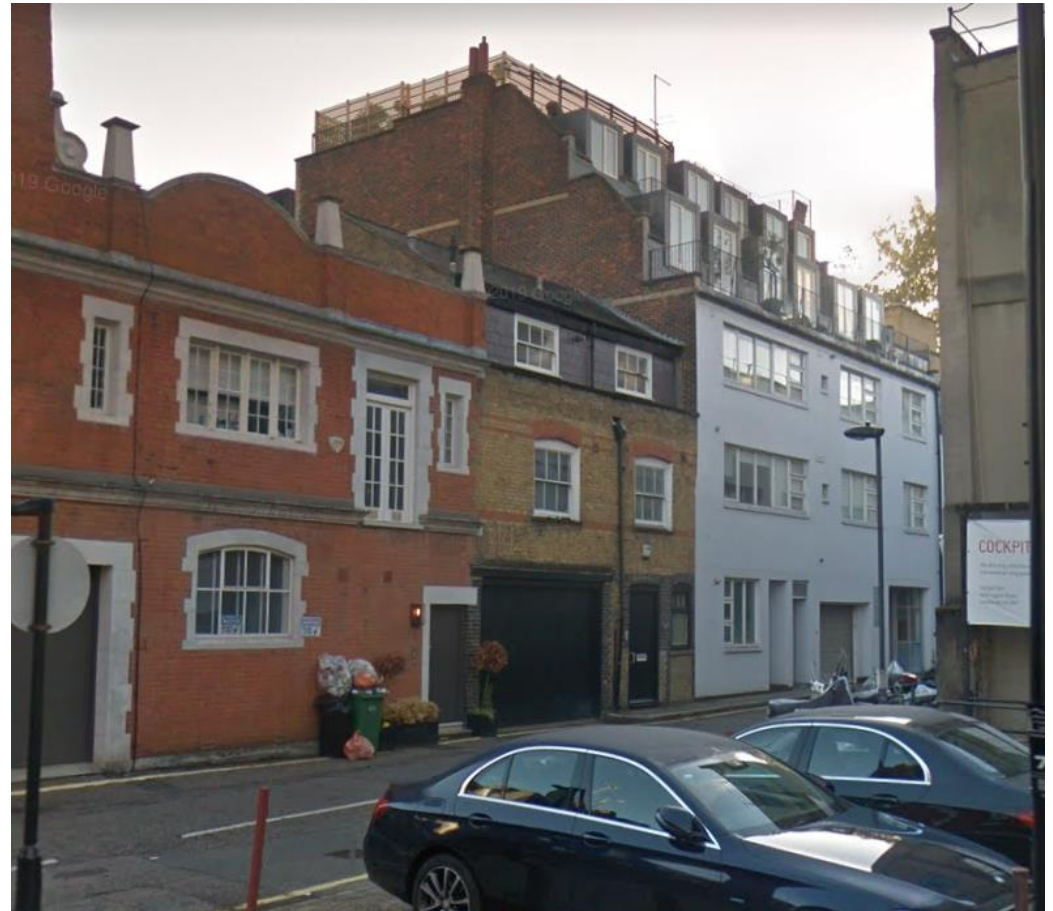
Photo 2 (above): Street view of application site
