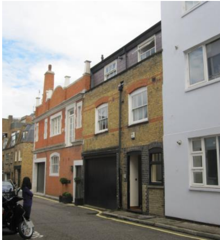
Figure 1: The existing site
