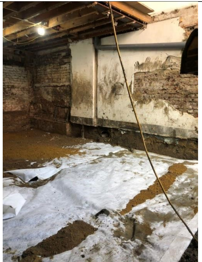
Geotextile membrane and new hardcore
