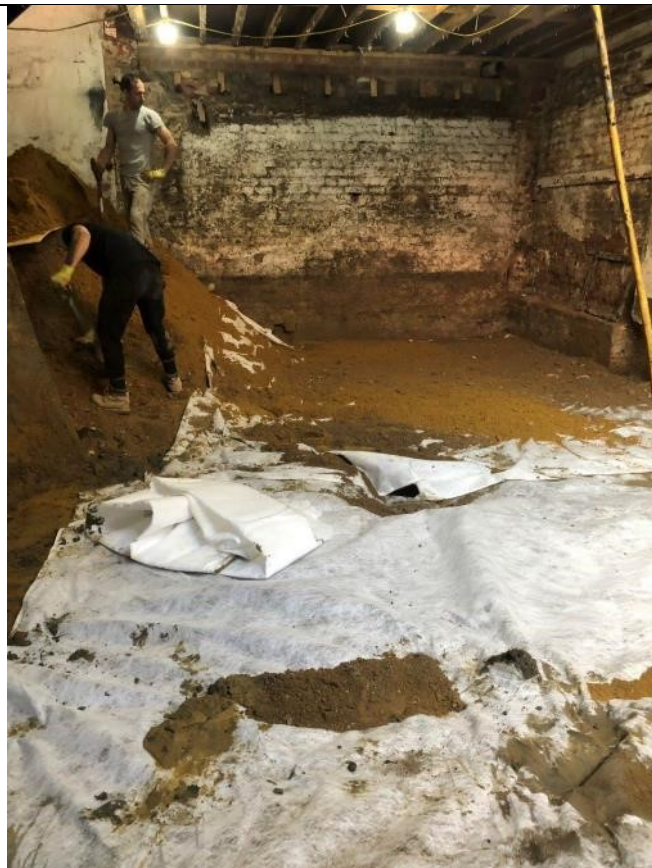
Geotextile membrane and new hardcore
