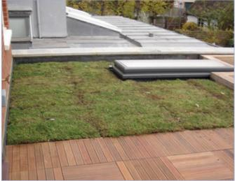
The modular sections mean detailing around objects is a simple process and clean lines are created. Hard landscaping sections such as paving and decking, mounted onto Wallbarn pedestals, can be added to the area to allow for regular access. As everything is suspended on top of the deck, drainage is uninterrupted.
