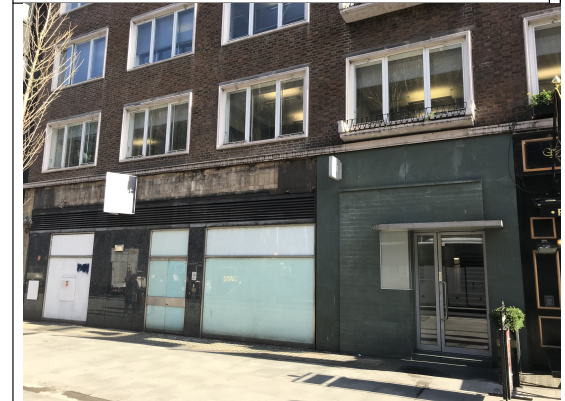
Photo of Existing External Elevation
