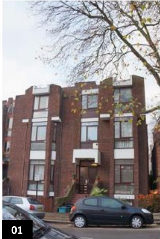
North Elevation viewed from Hampstead Hill Gardens
